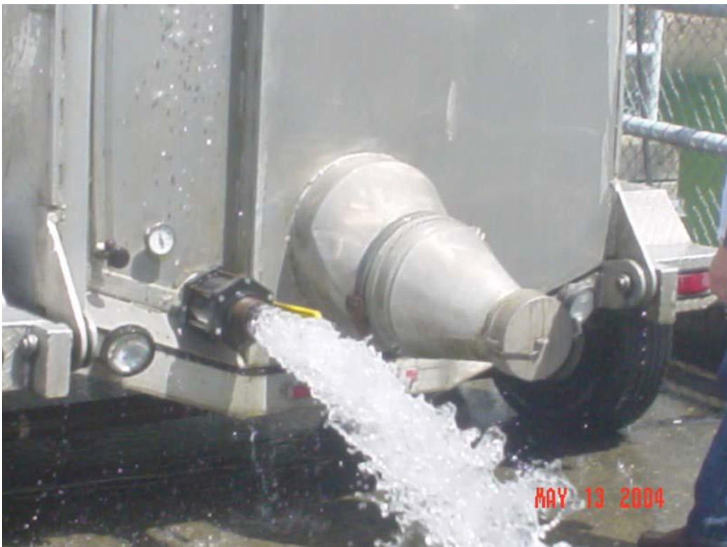
Figure 4 Drain Valve and Release Pipe
