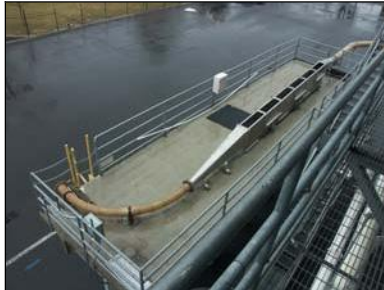
Truck Loading Facility
