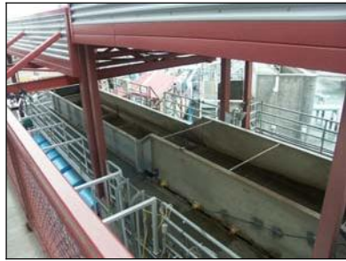
Separator Looking D.S.
