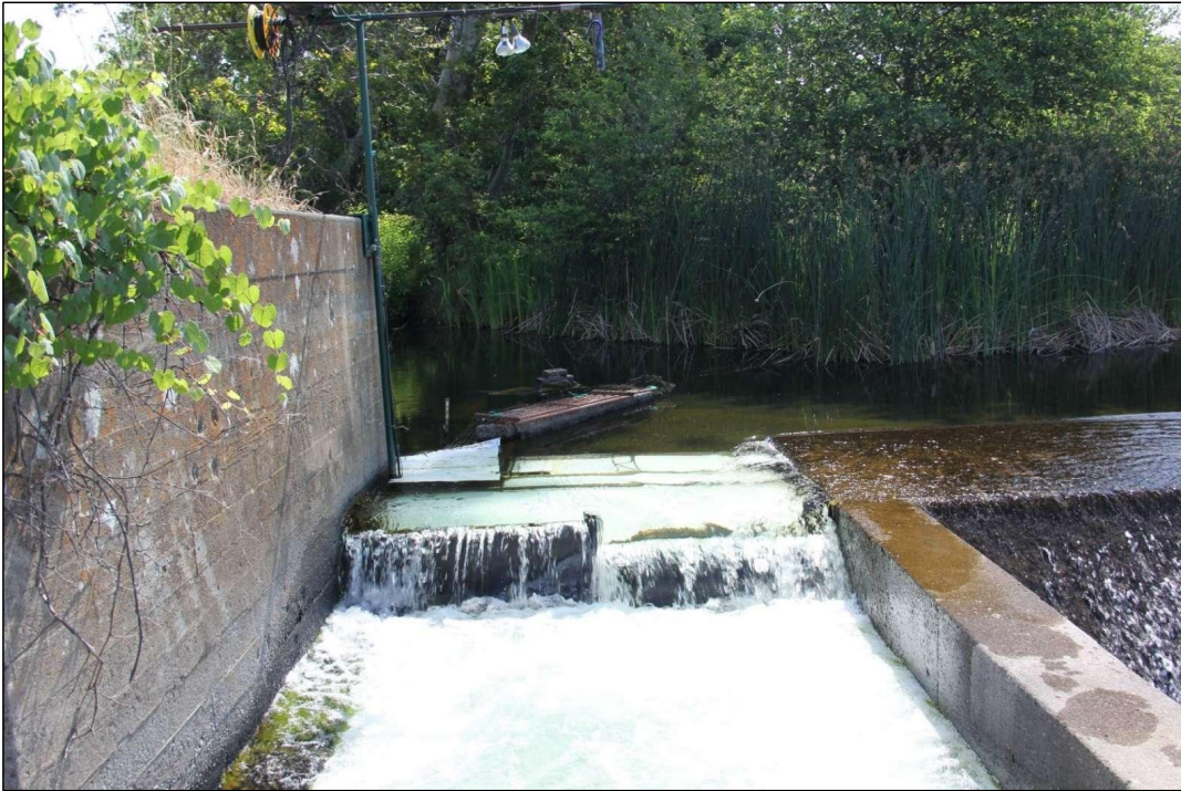
Appendix F Figure F20. The Deer Creek North video station in at the top of the fish ladder at Stanford Vina Dam.
