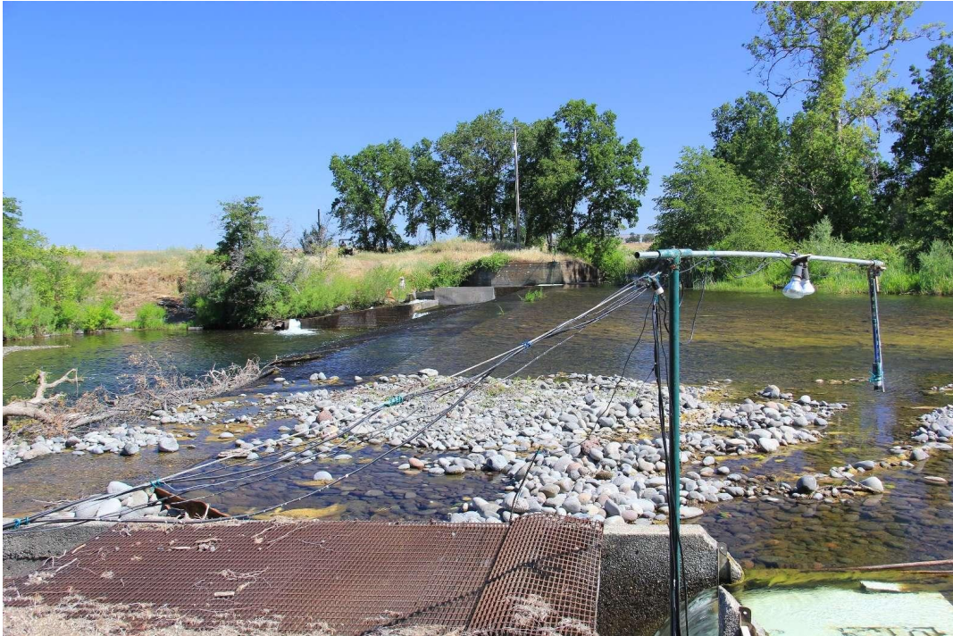
Appendix F Figure F19. The Deer Creek South video station in 2016 at the fish ladder at Stanford Vina Dam. The North station is visible in the distance across the dam.
