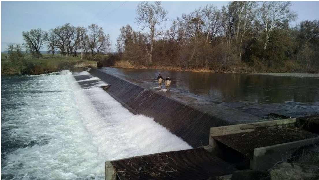
Appendix F Figure F21. The RBFO video crew cleaning the Deer Creek video stations at Stanford Vina Dam.
