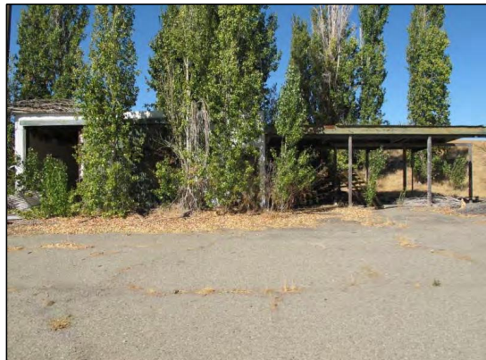
Photo 4. View of former hazardous materials storage area facing west. No current hazardous materials were observed.
