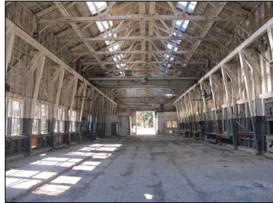
Photo 2. Interior of the former ship repair shop facing south.
