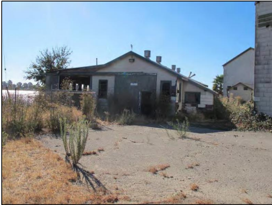
Photo 1. View of former carpenter shed, electrical shop, and battery storage building facing south.
