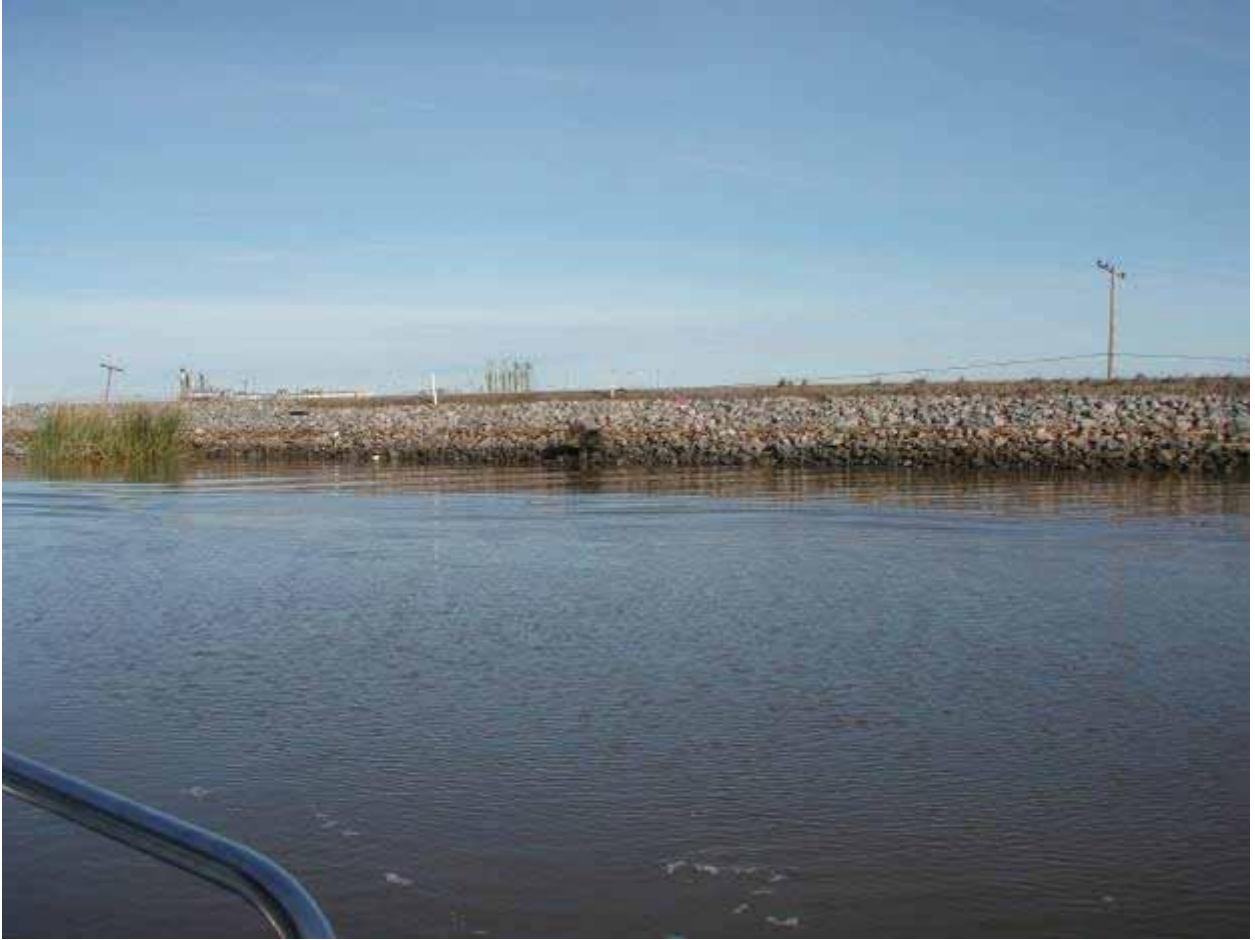
Figure C-5 - McDonald Island, with PG&E gas storage facilities behind levee
