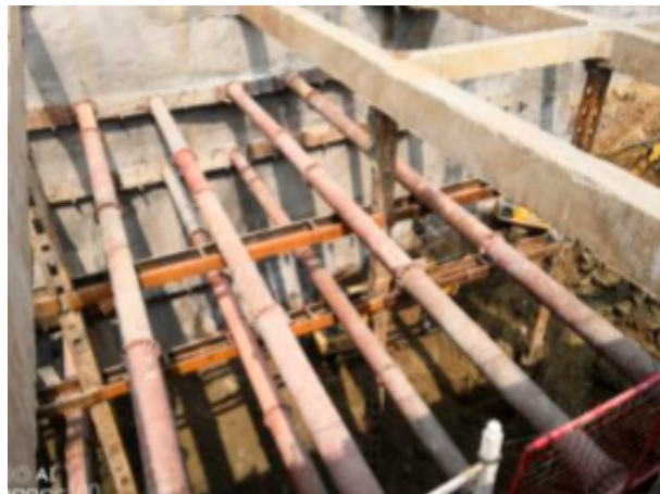
Figure 15. Steel support erection.
