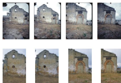
Figure 8 Two UMK 1318/10 stereopairs (above) and two Canon D30, with 20 mm lens (below), in the façade of St. Domingo de Silos' Church.
