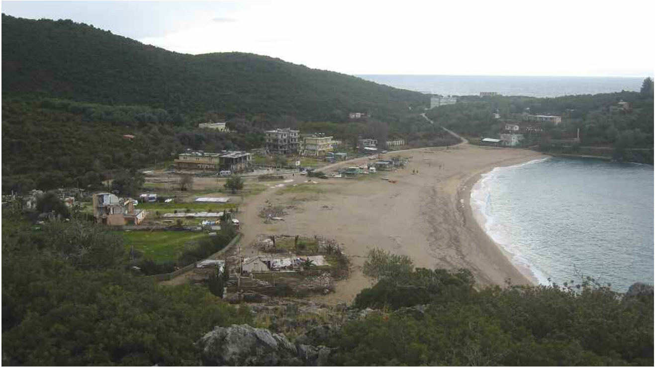
Demolitions at Jala (Jala Beach)
