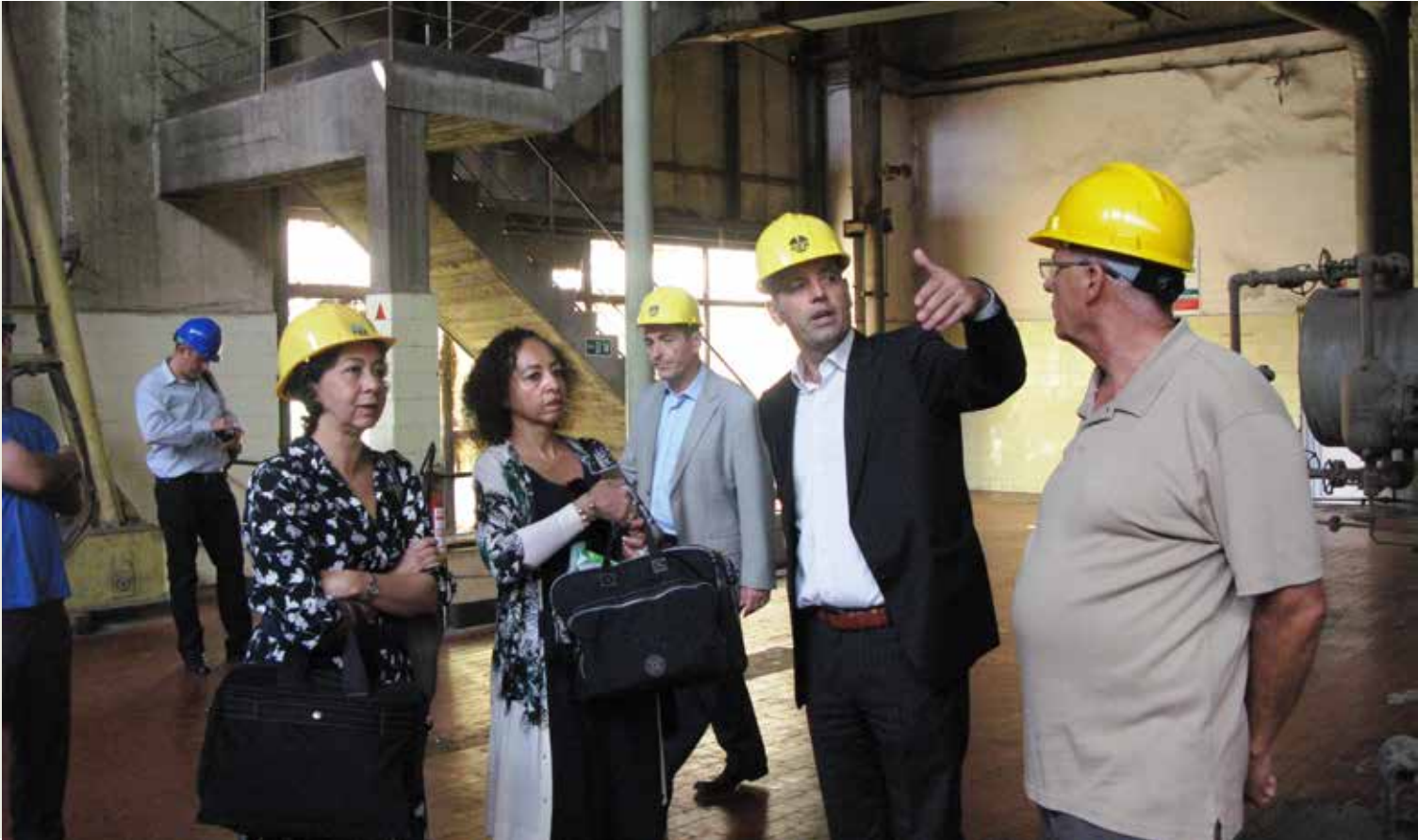
Panel Members visiting power plant in Obiliq, Kosovo
