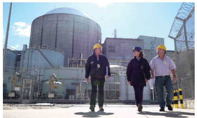
200th OSART mission in Almaraz Nuclear Power Plant, Spain
