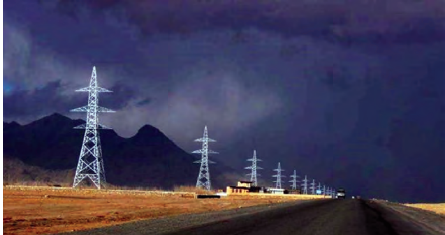
Transmission towers along the Arghandi-Ghazni line, part of more than 500 km of USAID-supported construction to connect power systems from Kabul to Kandahar and Helmand. (USAID photo)
