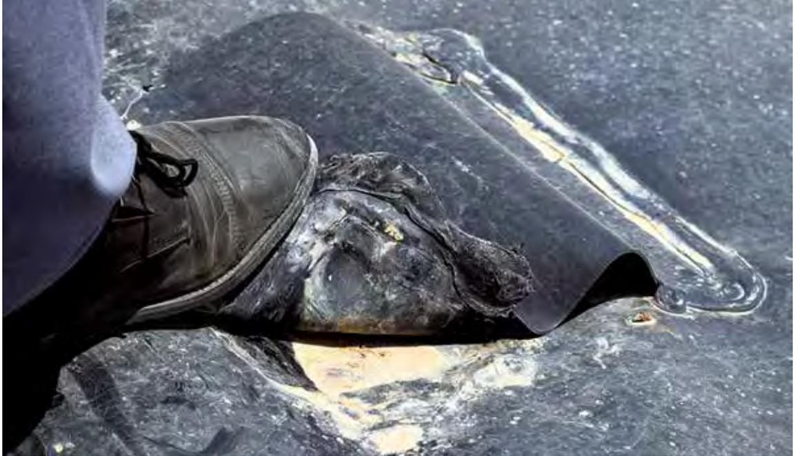
Detached pond liner air vent at a wastewater treatment facility. (SIGAR photo)
