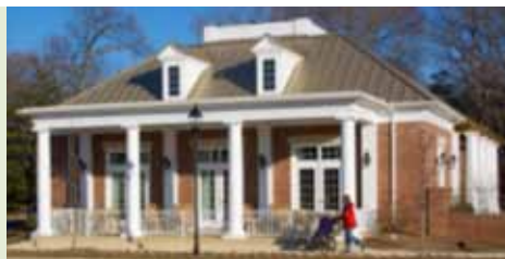
Fairfax Neighborhood Center, Fort Belvoir, VA.
