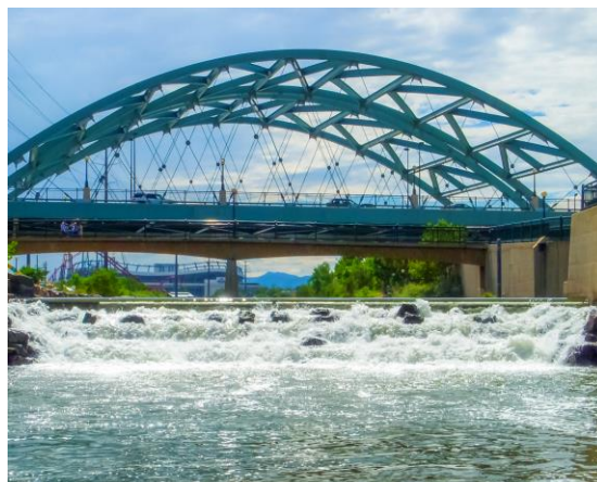
Figure 1: Mitigation in Confluence Park, Denver, Colorado
