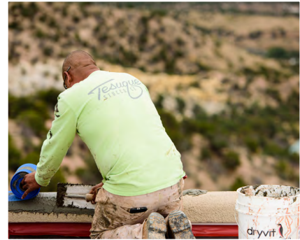
parapet repair
