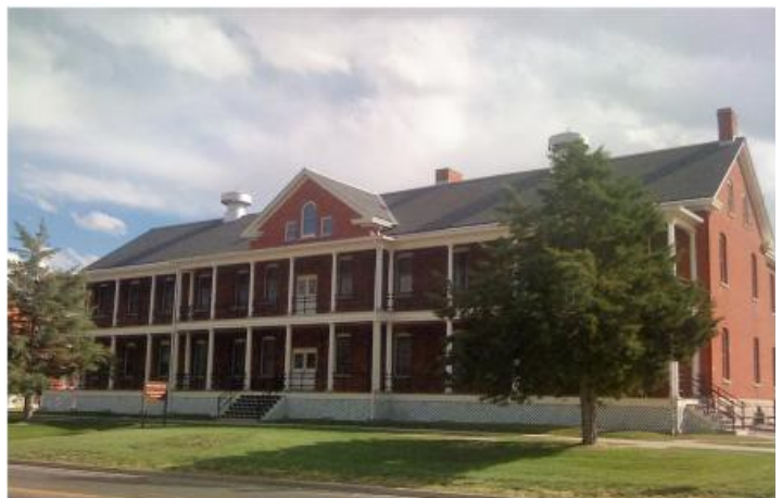
One of the Enlisted Men's Barracks, Building 222 at Warren Air Force Base, WY, was constructed between 1905 and 1910.
