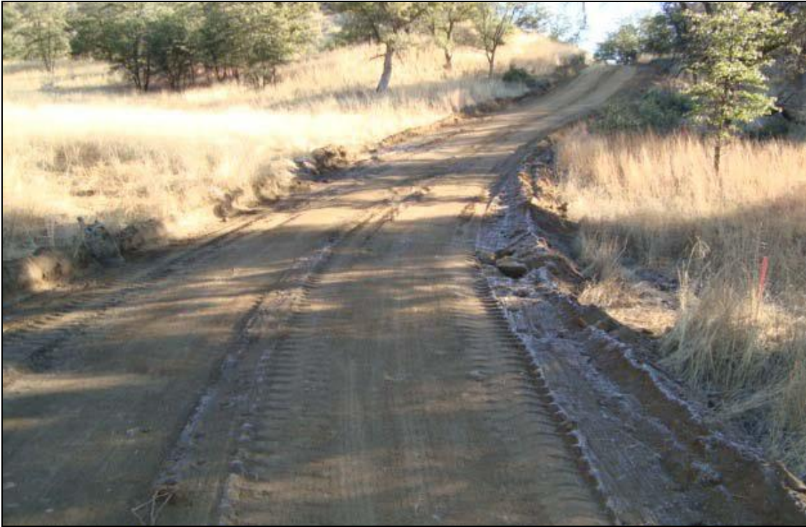
Figure 3-3. Photograph of Access Road for Section EV-1B
