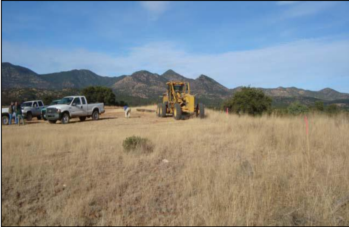
Figure 3-6. Photograph of Staging Area for Section EV-1B
