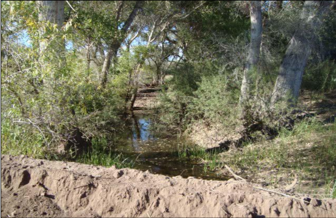
Figure 2-5. Photograph of Unauthorized Work in Black Draw in Section FV-1B
