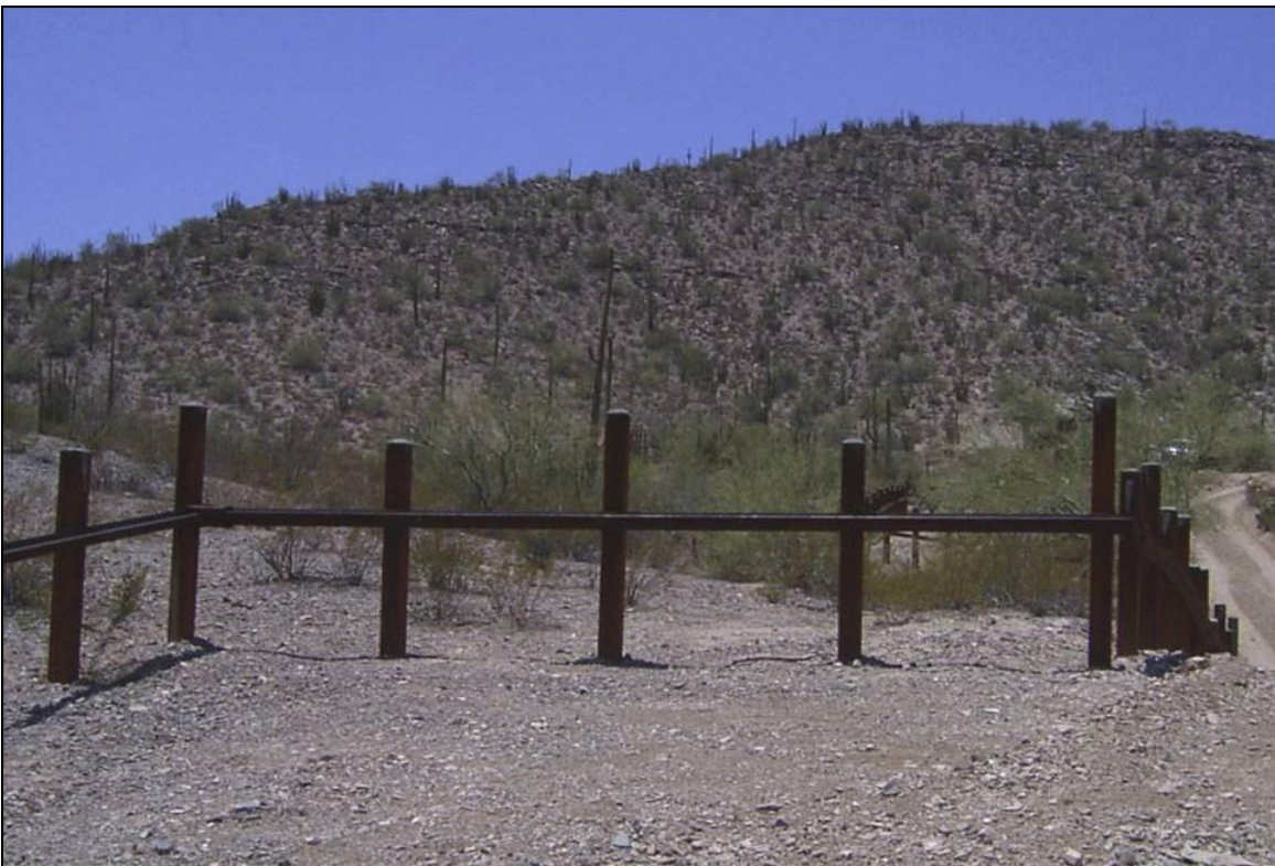
Figure 2-2. Photograph of Post-on-Rail Fence
