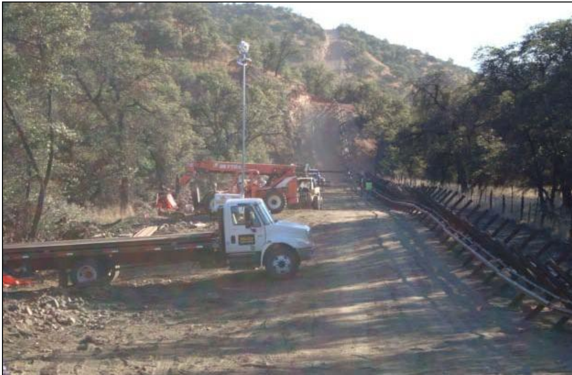
Figure 3-4. Photograph of Section EV-1B Fence Construction on Steep Terrain
