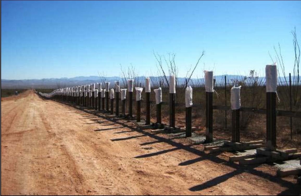
Figure 3-5. Photograph of Section FV-1B Fence Construction
