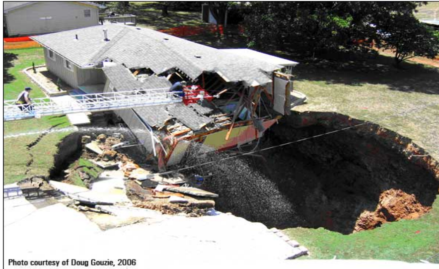
Figure 3.4-2. Sink Hole in Karst Topography
