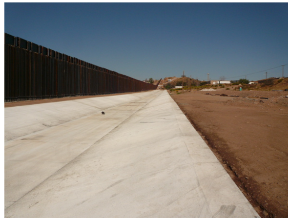
Photograph 1. Overview of the concrete-lined drain, west of Maricopa POE.
