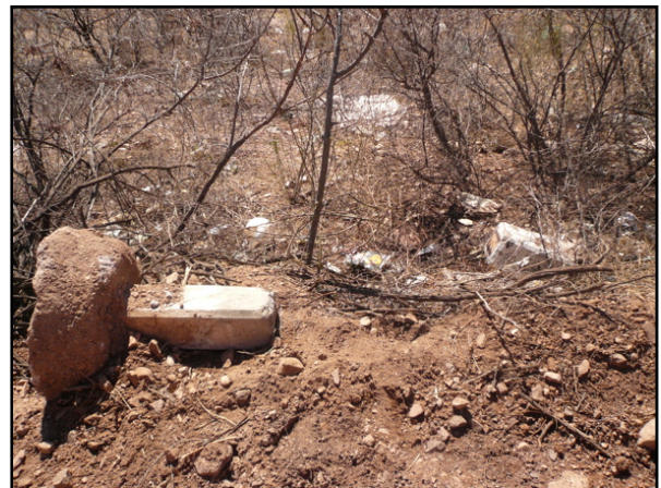
Photograph 4. Broken Border Marker IBWC 123, west of Mariposa POE.
