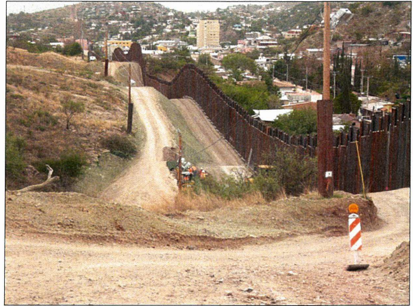
Photograph 6. Green hydromulch on hillside between elevated legacy road and new construction road, west of the DeConcini POE.
