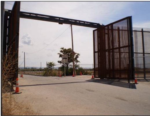
Photograph 3-9. Fabens POE Swinging Vehicle Gate Installed.
