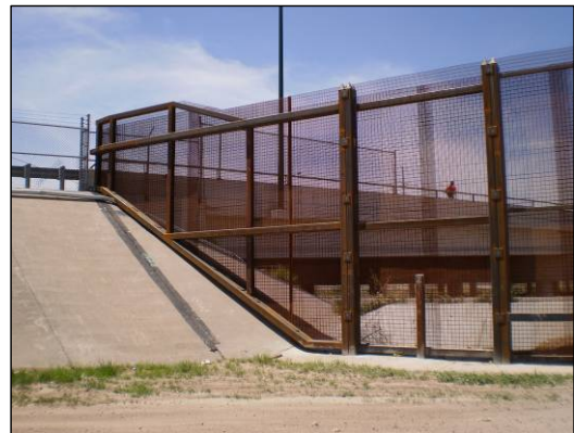
Photograph 3-1. Zaragoza POE Cantilevered Fenced Segment.
