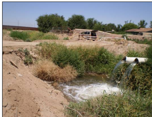
Photograph 3-5. Pompas Waste Canal Culvert Crossing.
