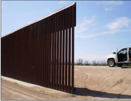
Photograph 3-11. Bollard Fence Installed in Segment K-5, West End.
