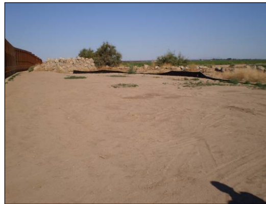
Photograph 3-10. Staging Area at the Fabens Waste Channel.
