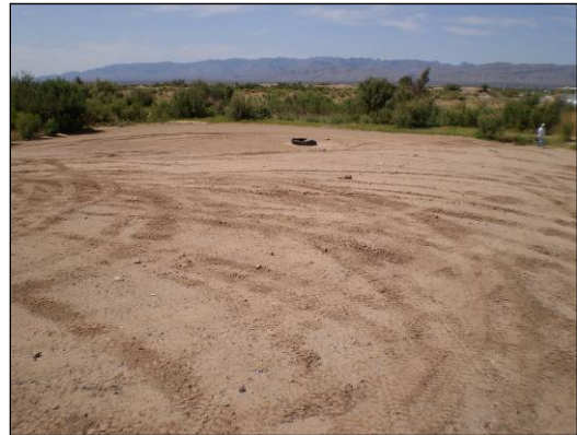
Photograph 3-13. Fort Hancock POE Staging Area.
