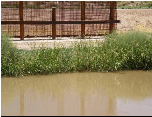
Photograph 3-2. Geo-Textile Canal Bank Stabilization.
