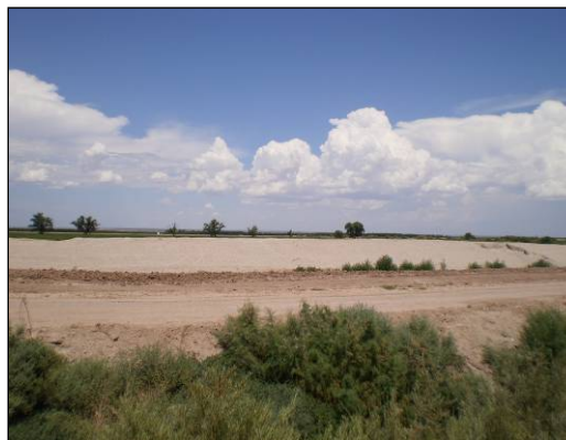
Photograph 3-8. Gravel Pile on Staging Area at TJ's Crossing.
