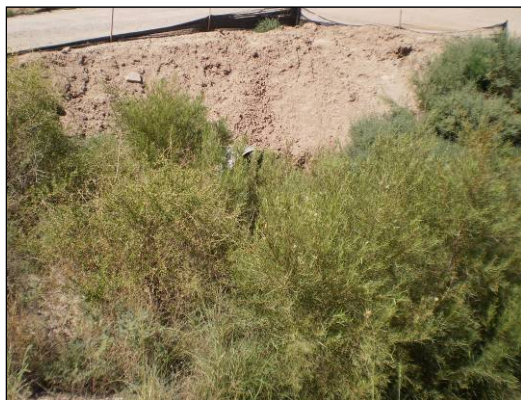
Photograph 3-7. TJ's Crossing Temporary Culvert Installed.
