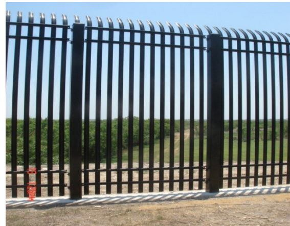
Photograph 3-1. Primary Pedestrian Fence with Aesthetic Quality
