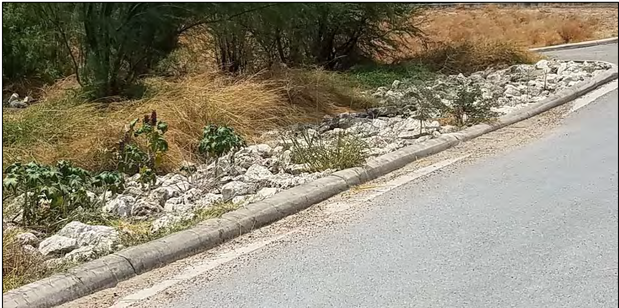
Figure 7-4. Typical Rip Rap Community consisting of large gravel rocks to control erosion.
