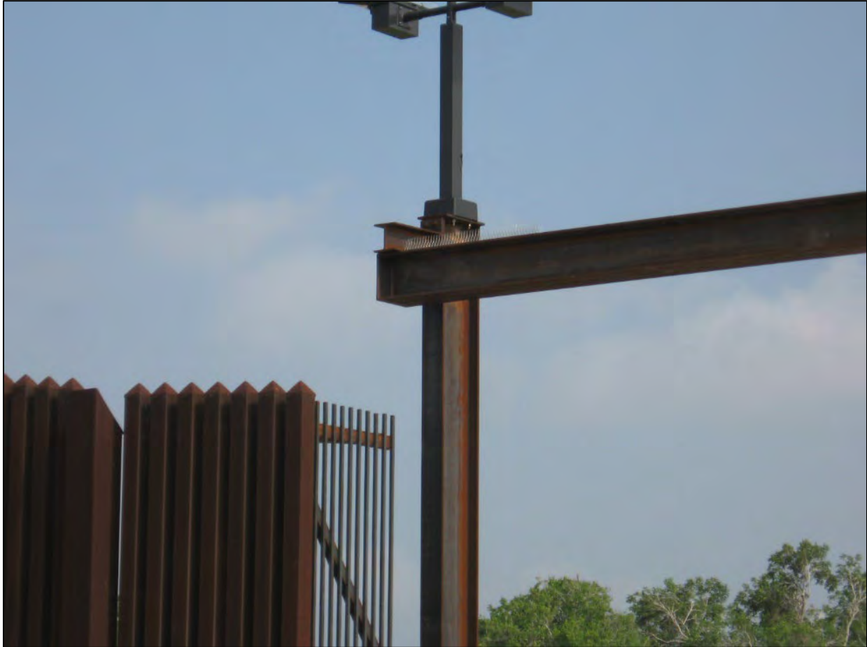
Figure 7-5. Bird Exclusion Devices along a gate in McAllen Sector.
