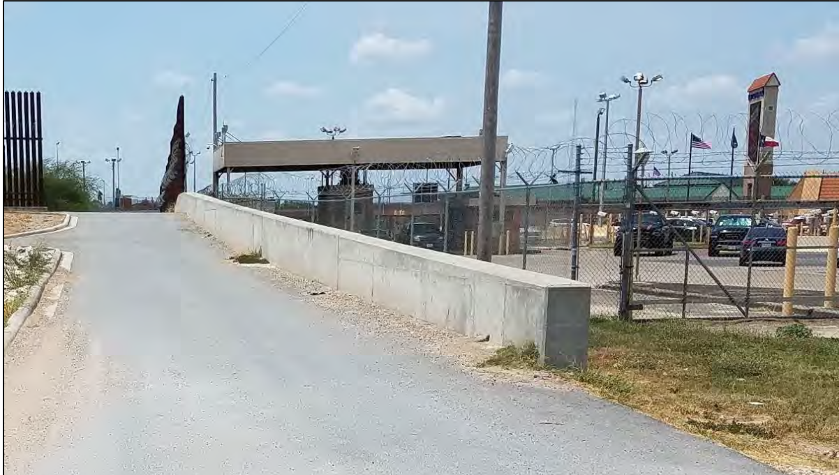
Figure 7-1. Typical Asphalt area
