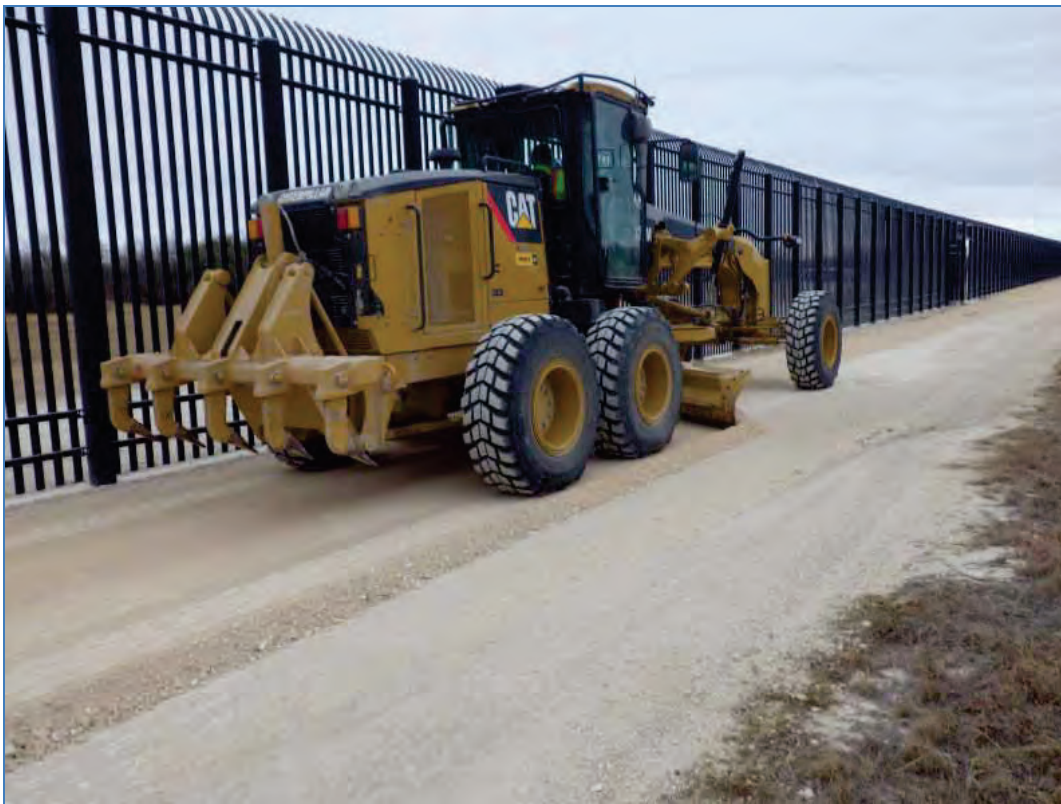
Figure B-11. Standard Grading Equipment
