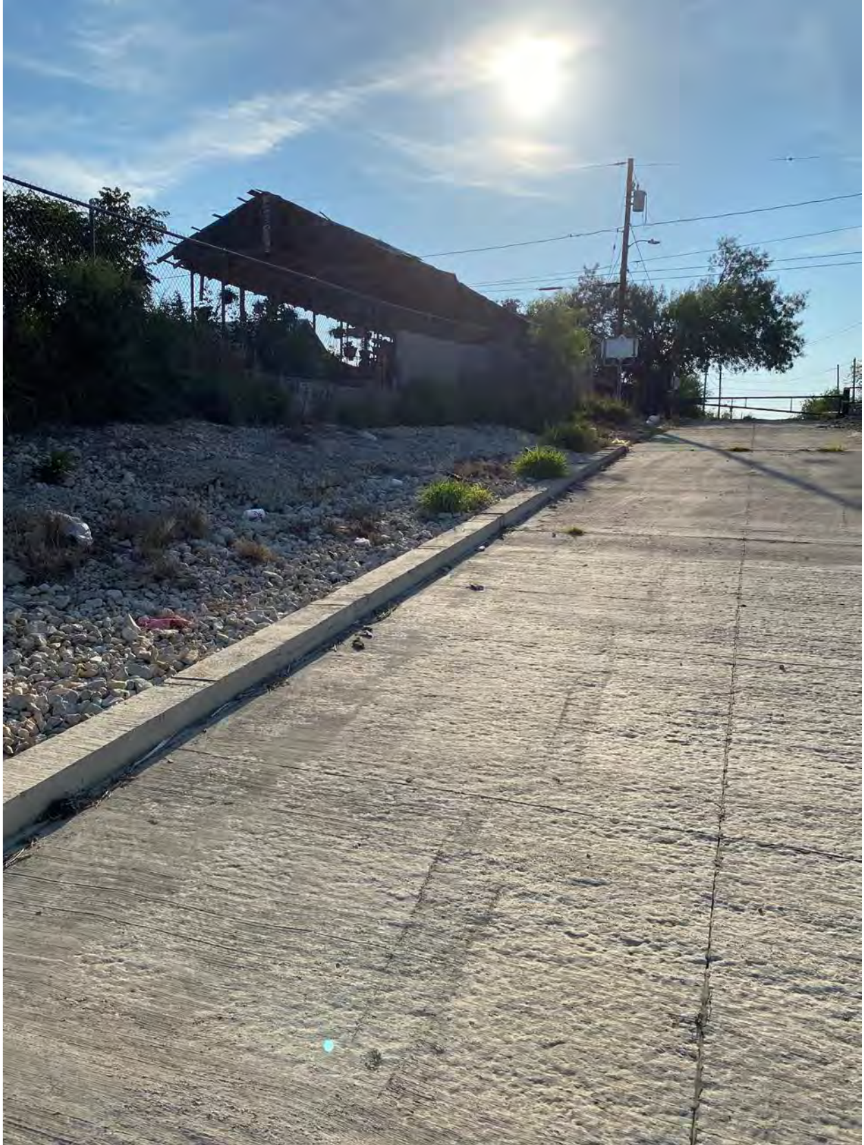
Photograph 51. Photopoint 16 – Facing East (See Figure A17)
