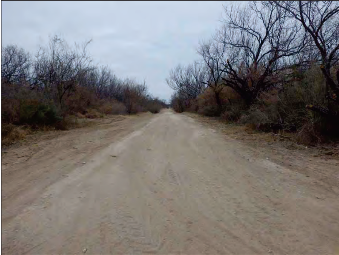
Figure B-5. FC-3 Graded Earth Road (Photograph)
