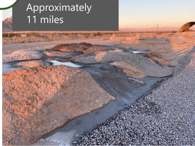
Right: Road work in El Centro Sector
