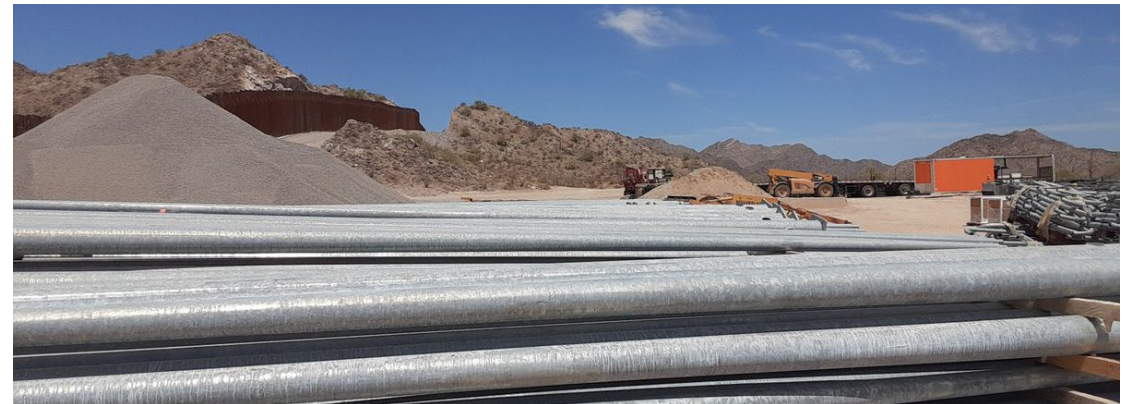
Below: Construction materials
