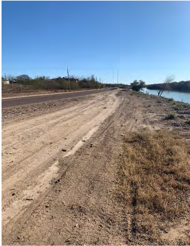
Figure 1-3. Current Project Area Conditions
