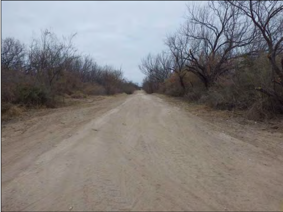
Figure A-5. FC-3 Graded Earth Road (Photograph)
