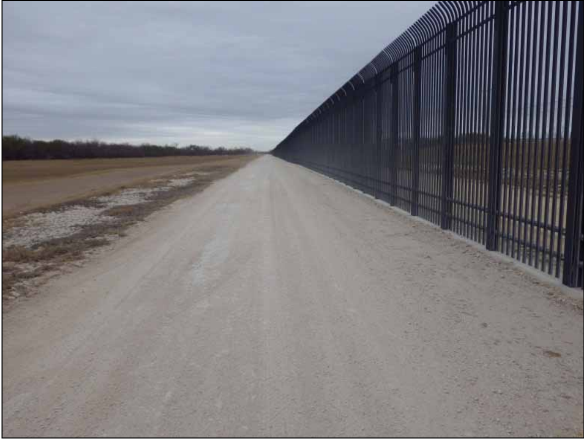
Figure A-3. FC-2 All-Weather Road (Photograph)
