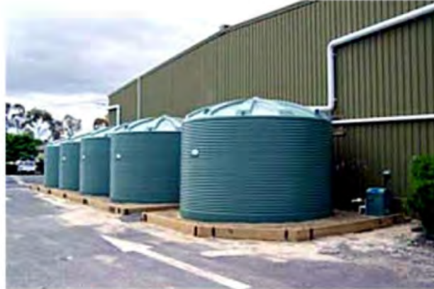
Figure 8a – Rainwater Harvesting in a Non-Residential Setting
