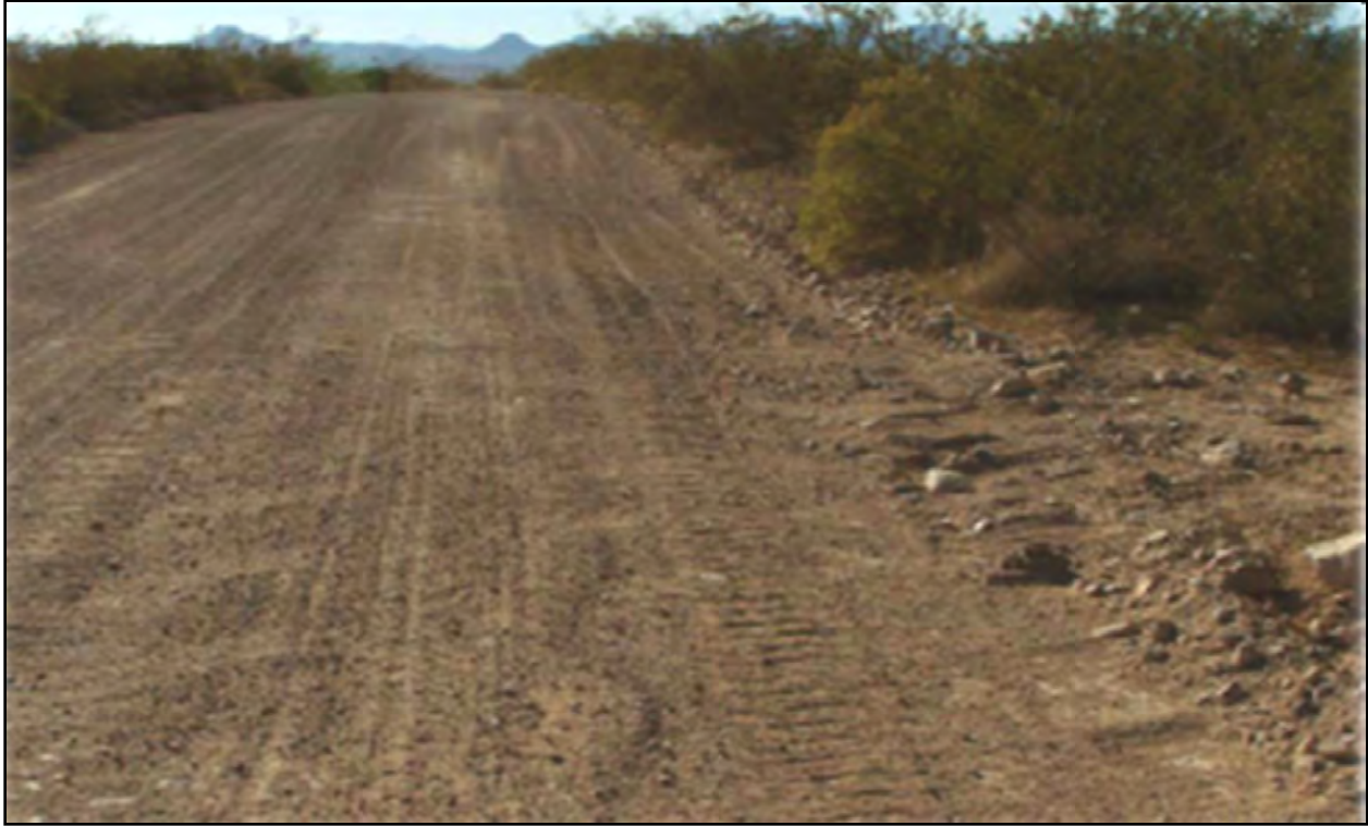
Figure A-5. FC-3 Graded Earth Road (Photograph)
