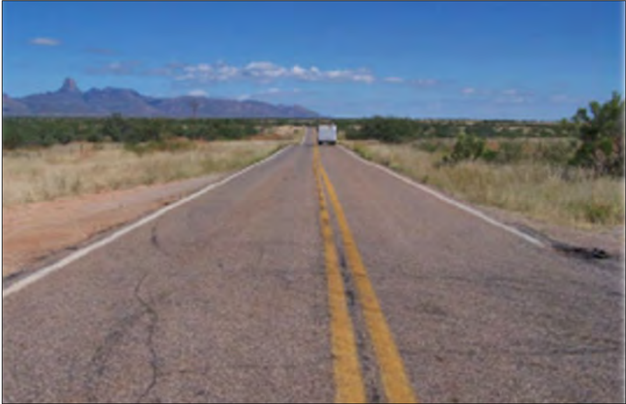
Figure A-1. FC-1 Paved Road (Photograph)
