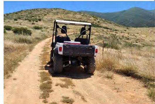
Water Cutout 9 (WC9)
