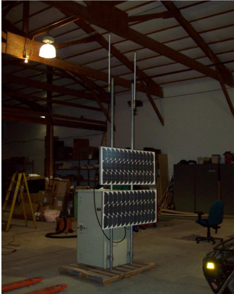
Enclosure 1: Representative Photographic of TCNS Shelter
