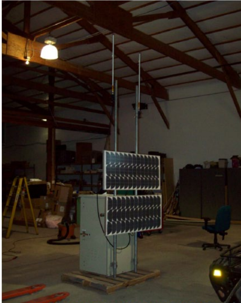
Enclosure 1: Representative Photographic of TCNS Shelter
