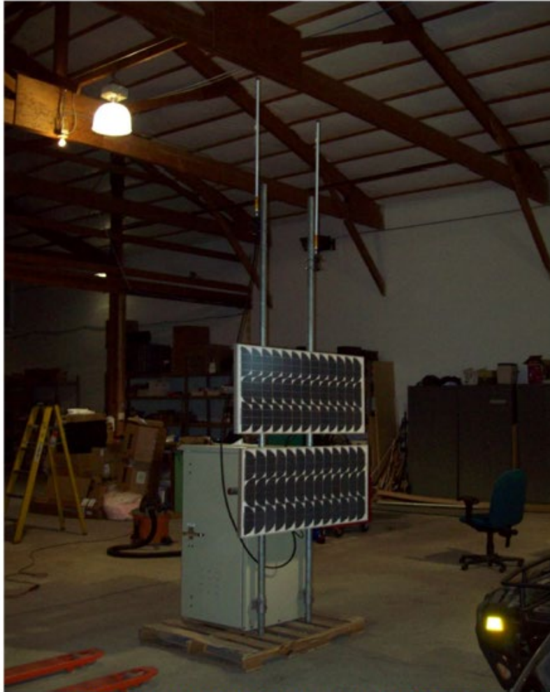
Enclosure 1: Representative Photographic of TCNS Shelter
