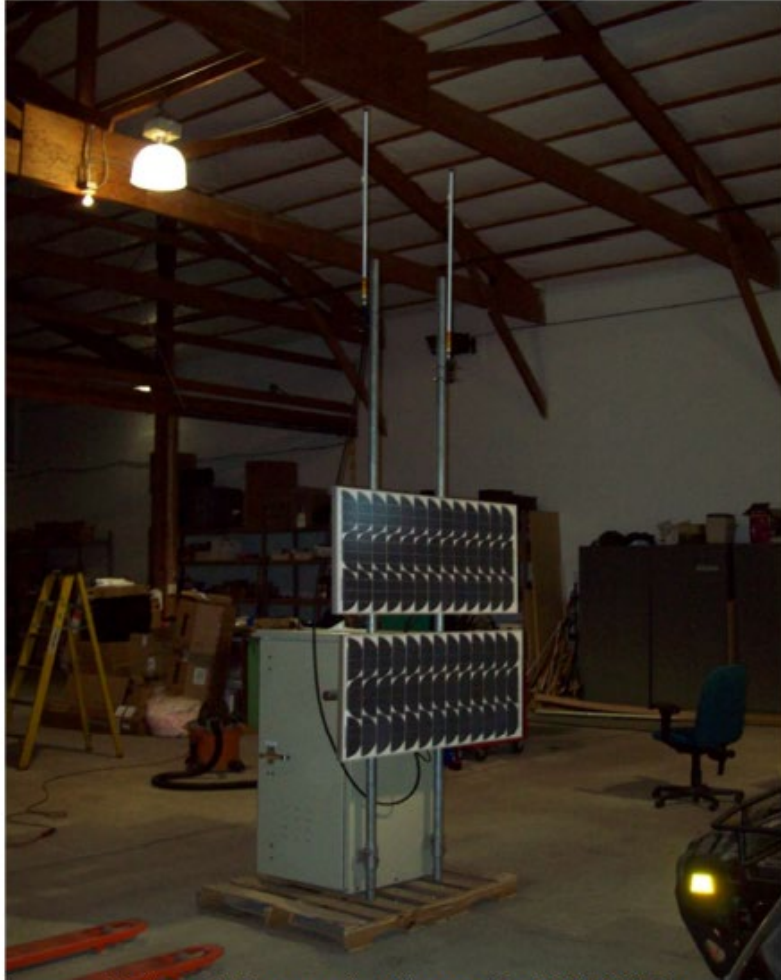
Enclosure 1: Representative Photographic of TCNS Shelter
