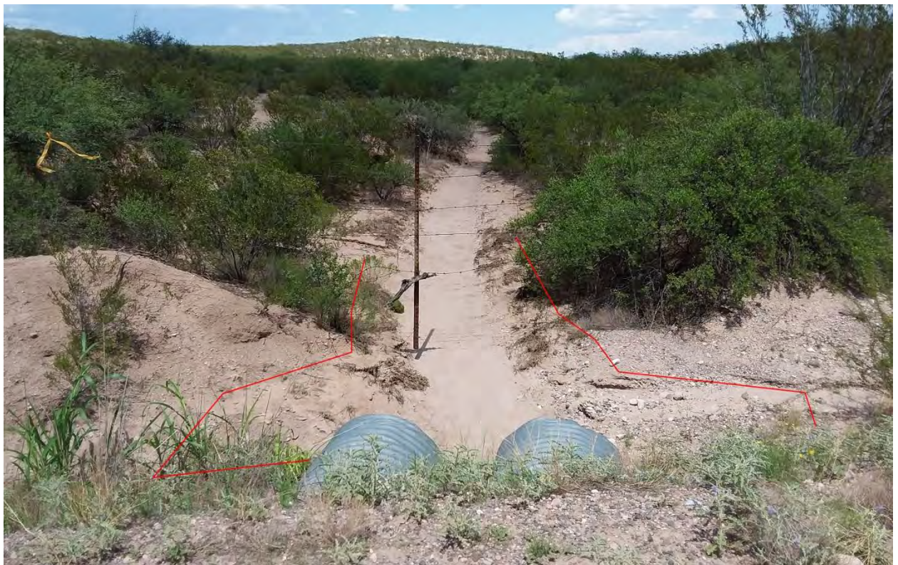
Figure 906. Photo point e9 looking upstream at culvert inlet.
