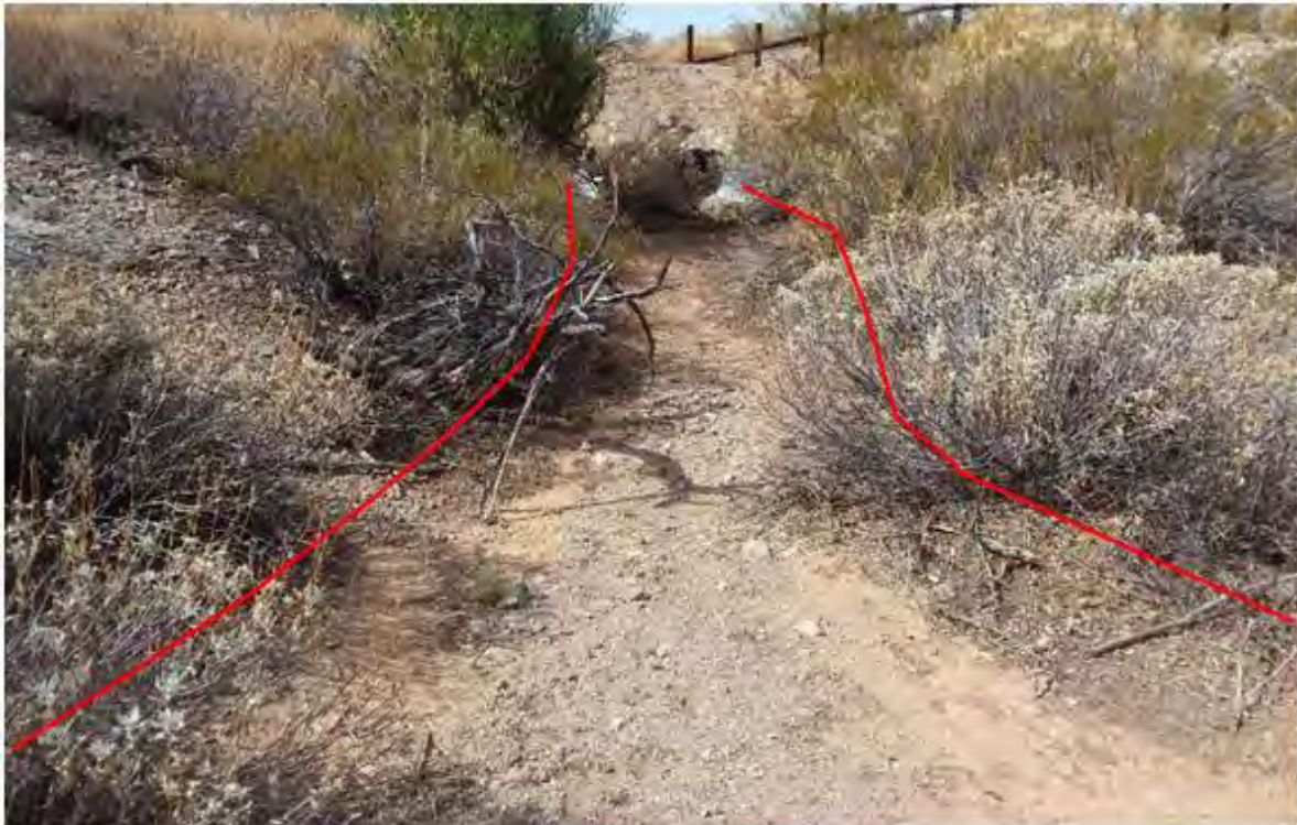
Figure 230. Photo point a17w3 looking downstream towards culverts
