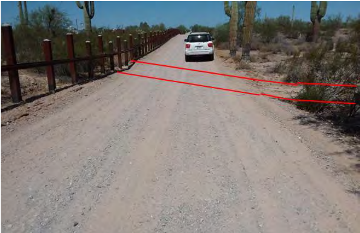
Figure 494. Photo point b9w10 looking west
