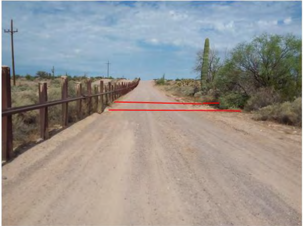
Figure 659. Photo point c1e1 looking west
