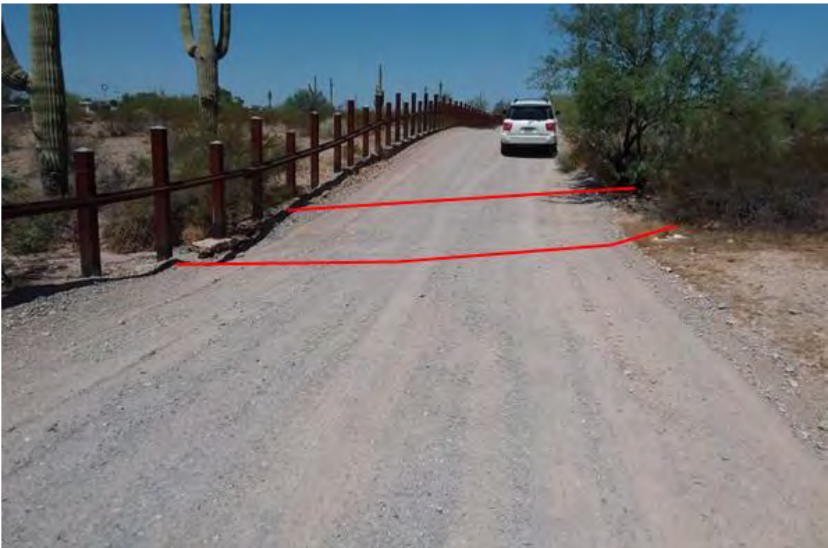
Figure 482. Photo point b9w15 looking west
