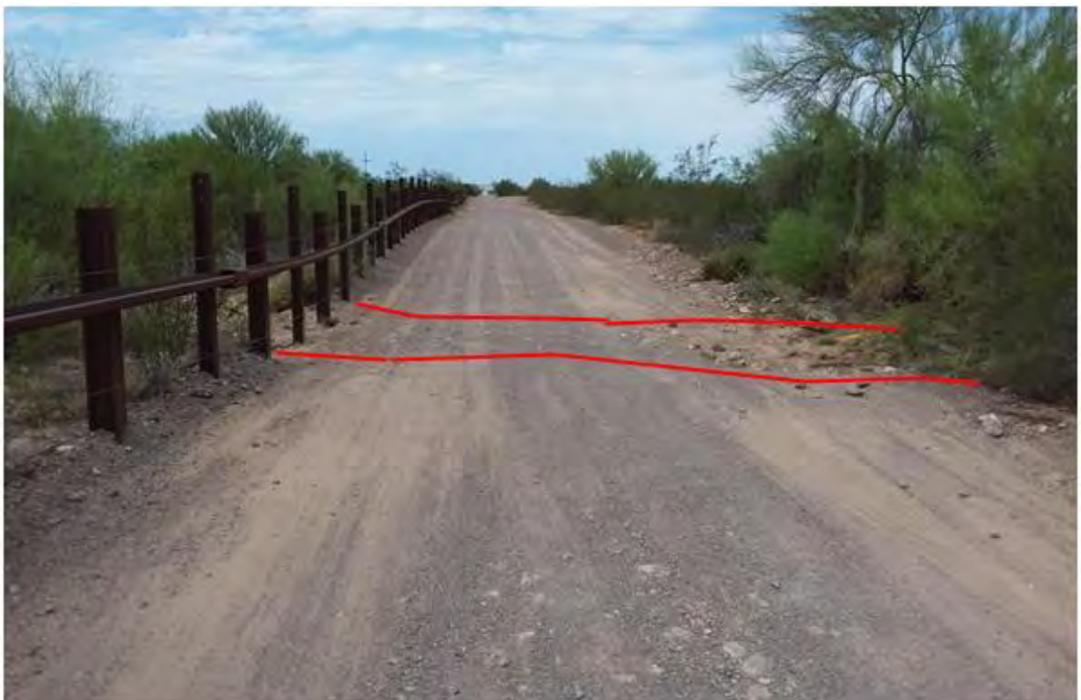
Figure 703. Photo point c4e5 looking west
