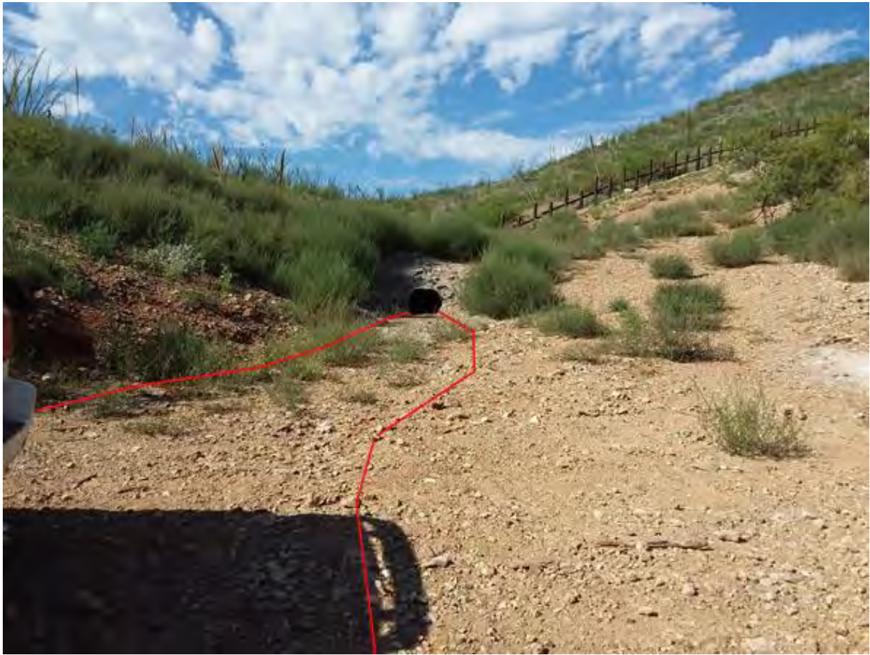
Figure 835. Photo point a13 looking upstream
