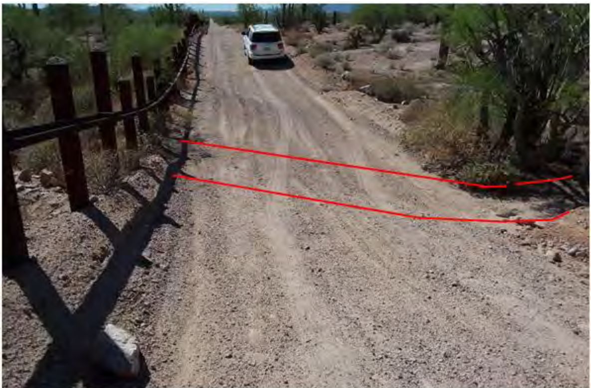
Figure 372. Photo point b1w2 looking west
