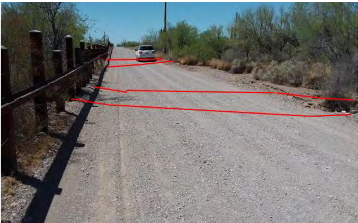
Figure 415. Photo point b3w2 looking west
