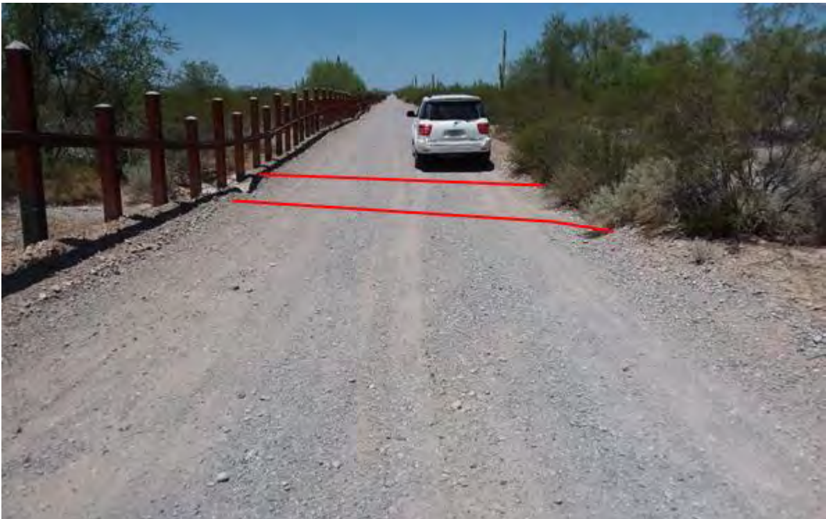
Figure 458. Photo point b7w2 looking west
