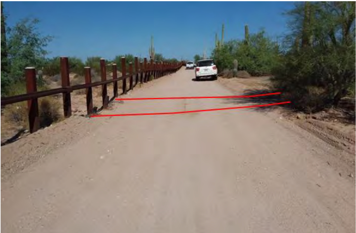
Figure 543. Photo point b10w4 looking west
