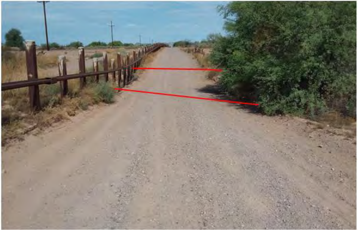
Figure 653. Photo point c0e4 looking west
