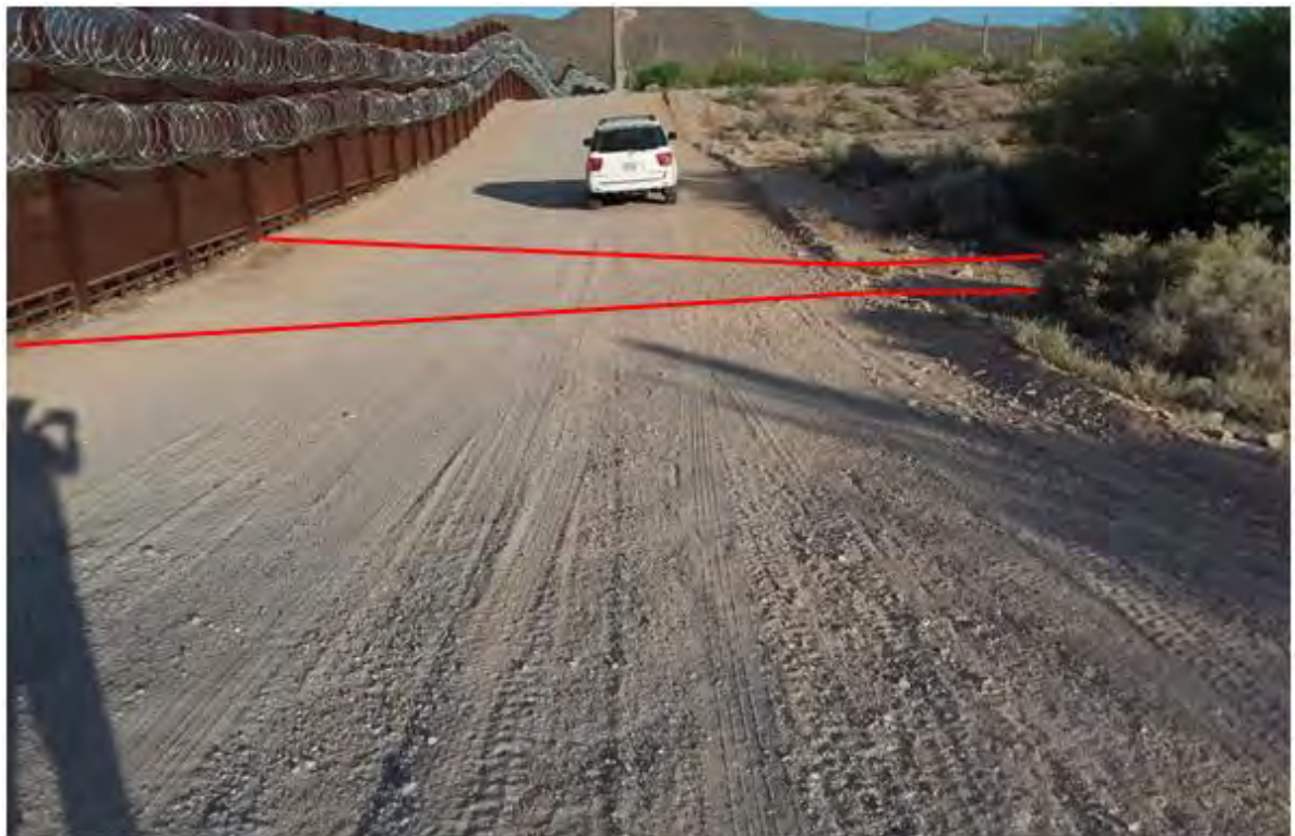
Figure 592. Photo point b15w2 looking west
