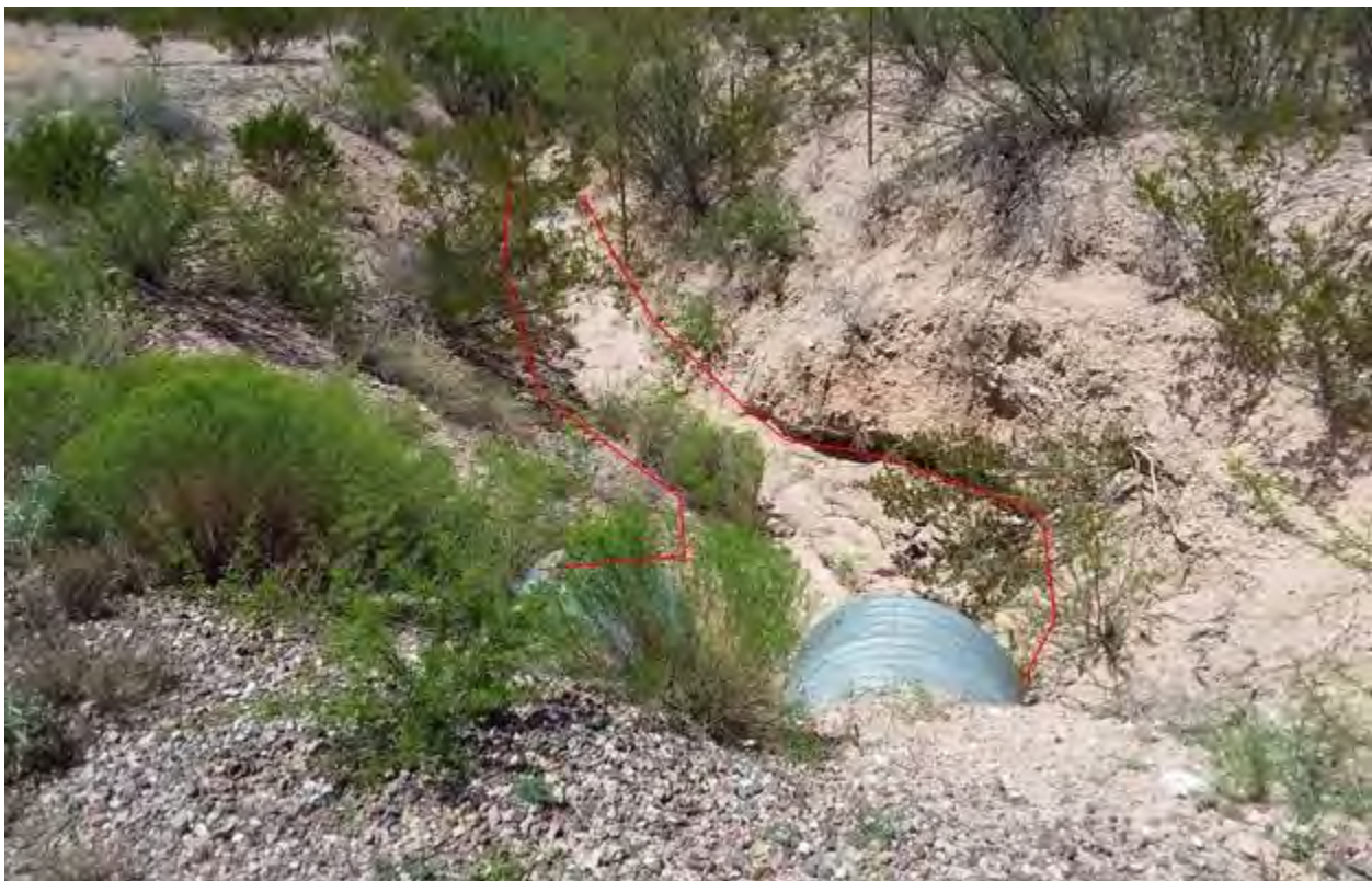
Figure 893. Photo point e6 looking downstream
