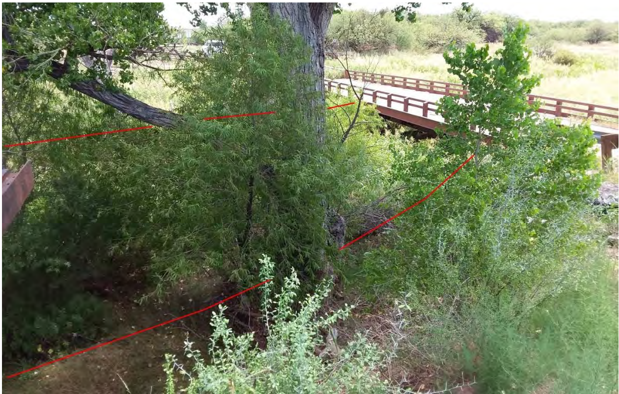
Figure 884. Photo point e2 looking downstream from the east bank
