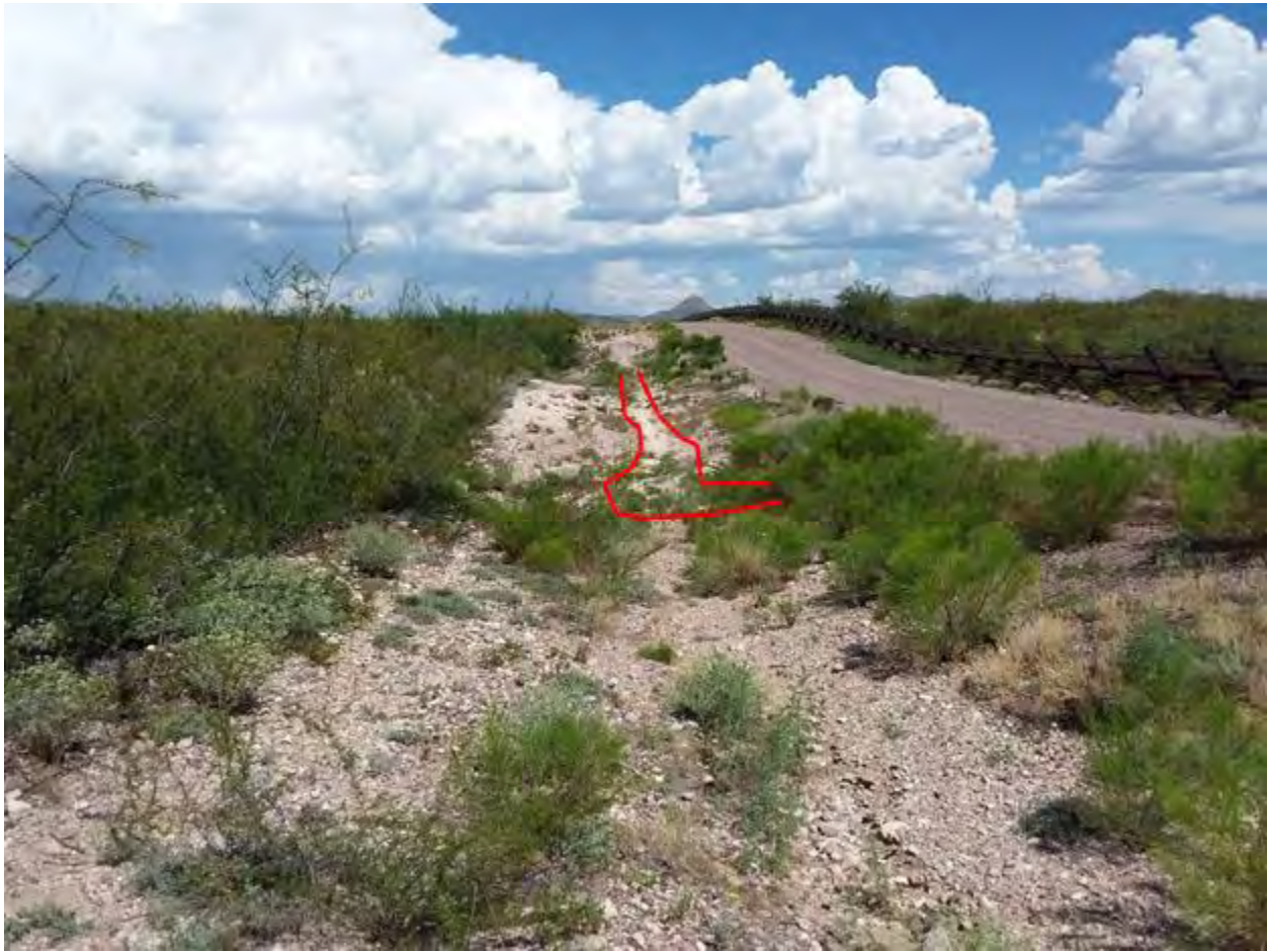
Figure 937. Photo point e24 looking east (flow crosses culvert under road)
