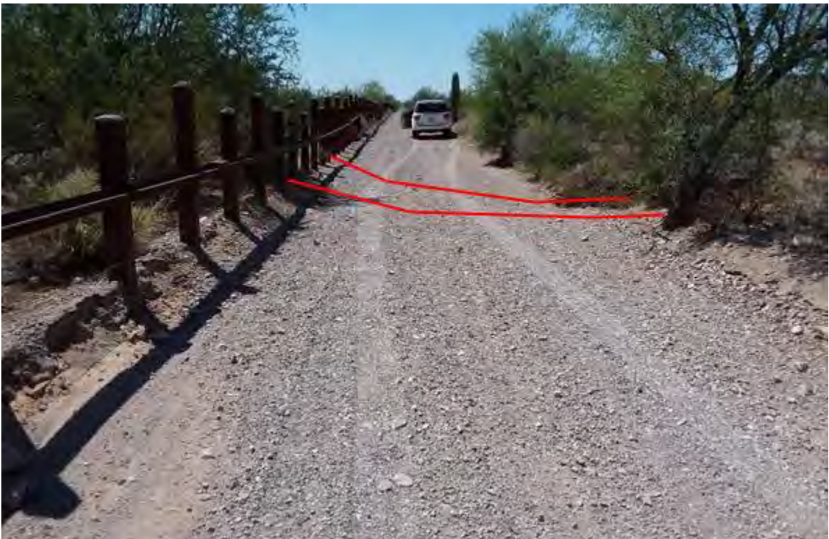
Figure 392. Photo point b3w10 looking west
