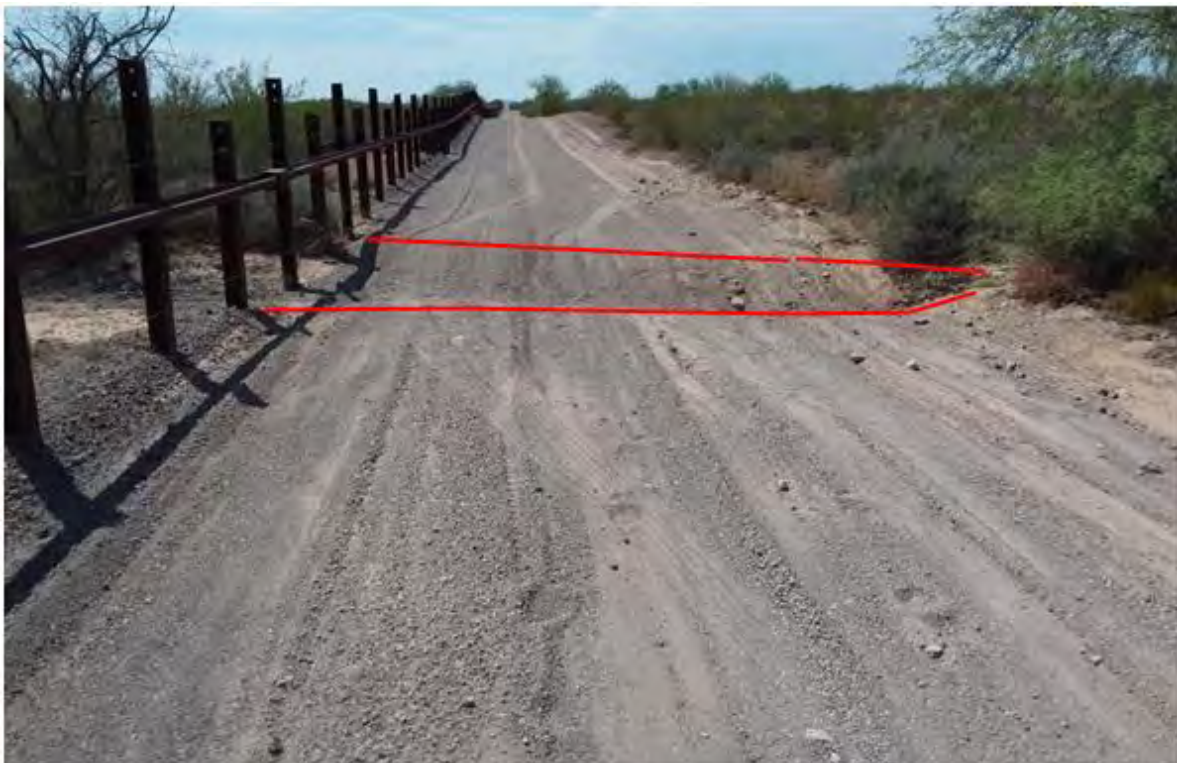
Figure 743. Photo point c5e3 looking west
