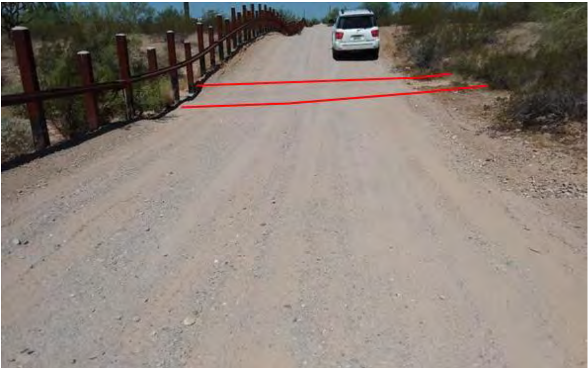
Figure 498. Photo point b9w8 looking west
