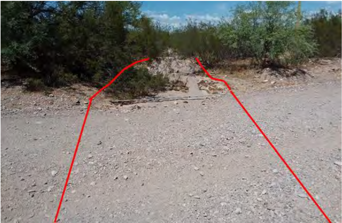
Figure 385. Photo point b3w11c looking upstream
