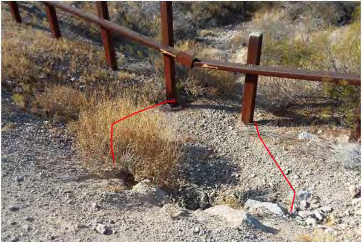
Figure 269. Photo point a22w4 looking downstream from culvert outlet
