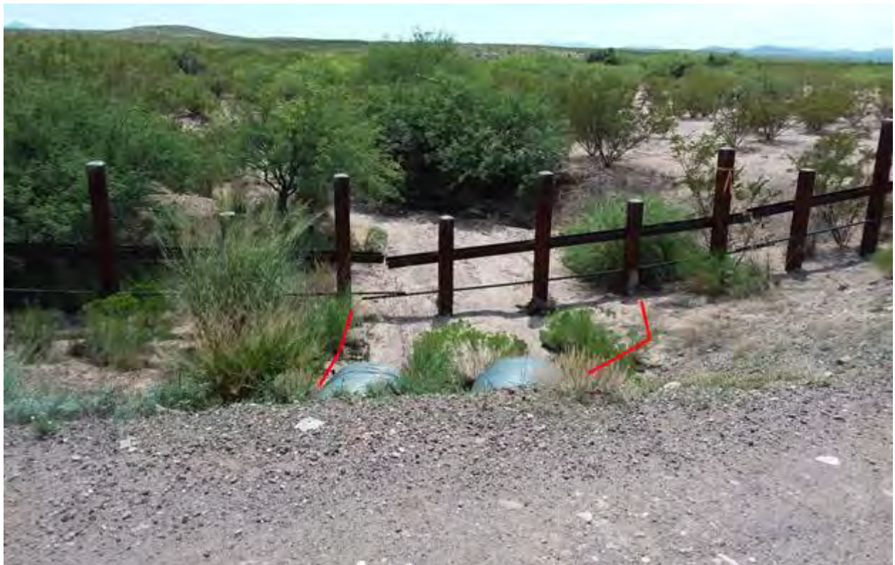
Figure 905. Photo point e9 looking downstream at culvert outlet
