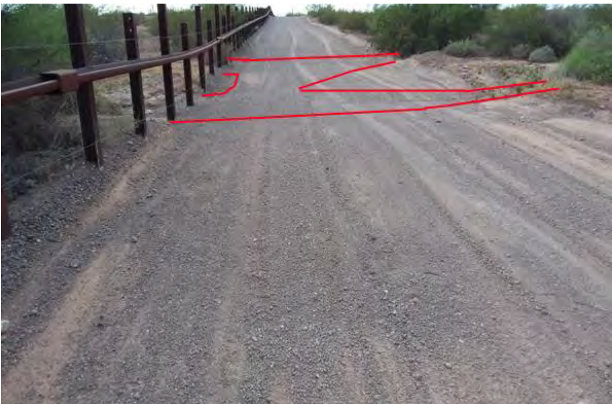
Figure 765. Photo point c6e6 looking west
