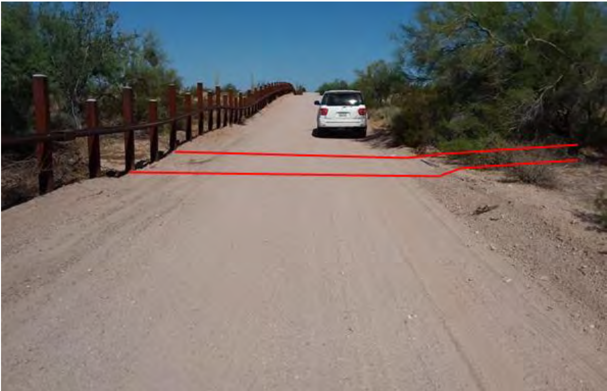
Figure 534. Photo point b10w7b looking west
