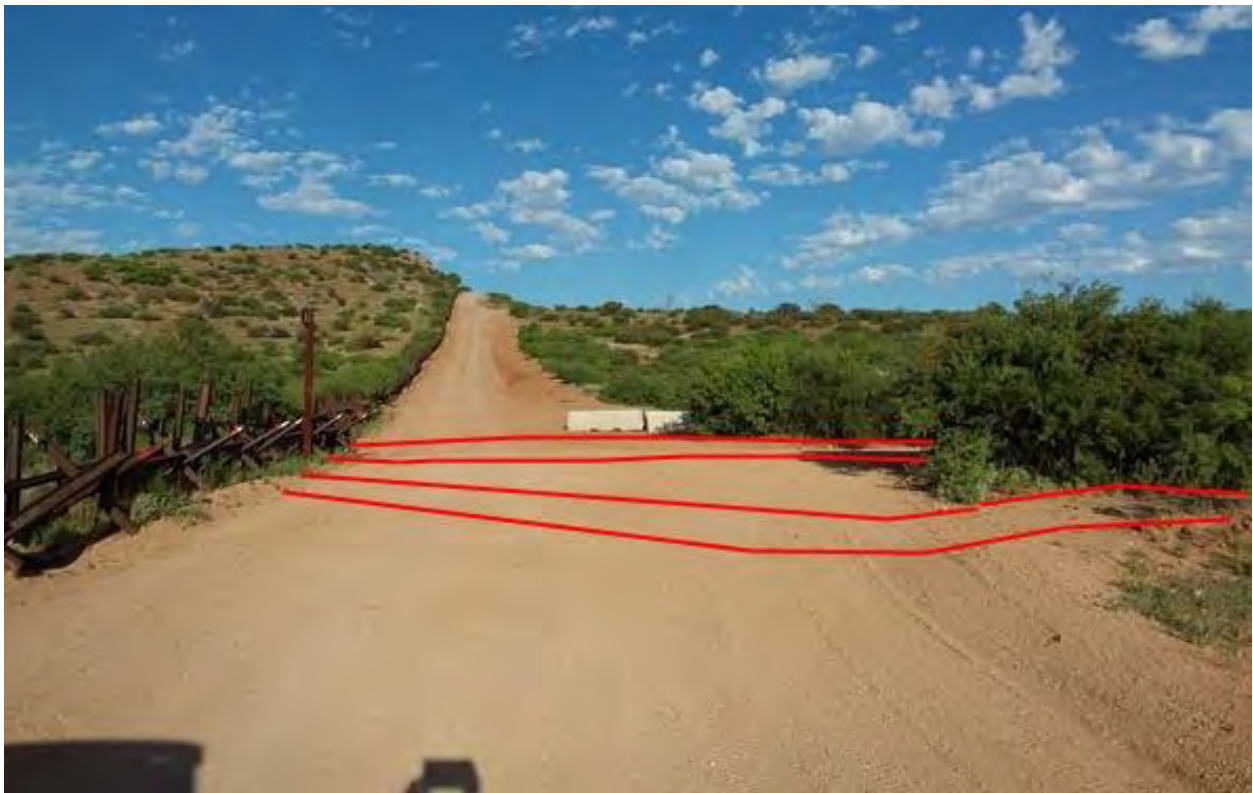
Figure 803. Photo point c1a looking west
