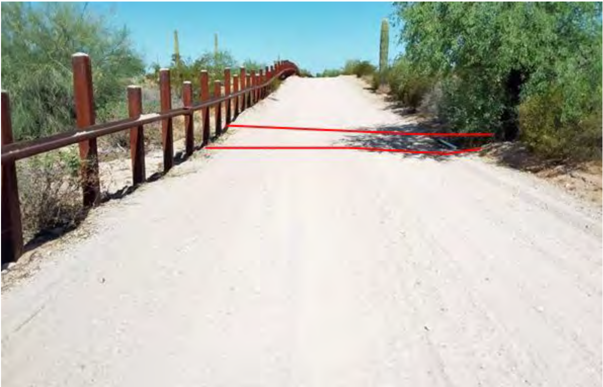
Figure 527. Photo point b10w10 looking west
