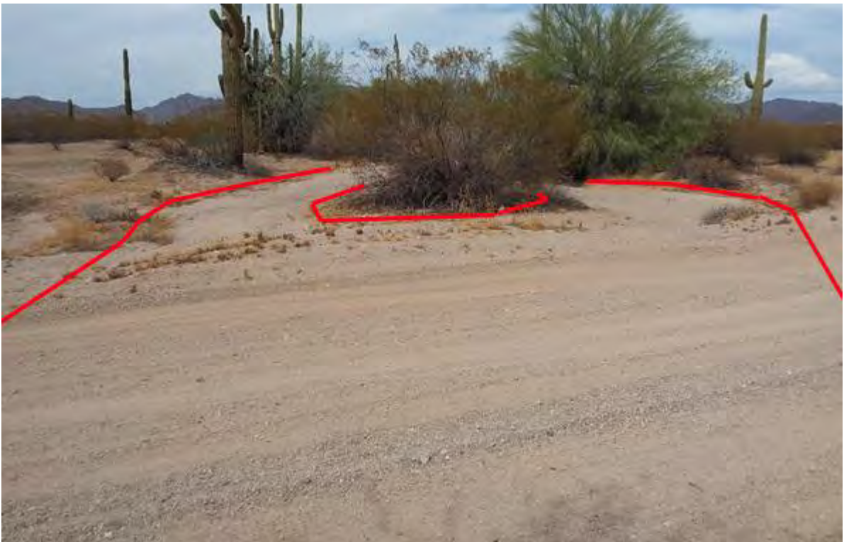
Figure 17. Photo point a2 looking upstream
