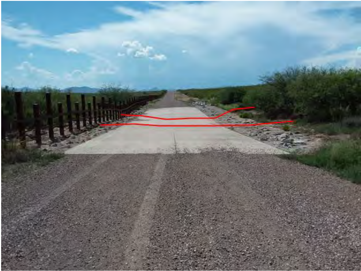
Figure 942 . Photo point e26 looking west
