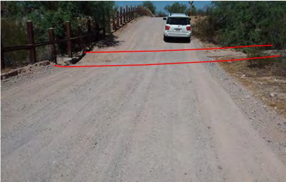
Figure 490. Photo point b9w11 looking west
