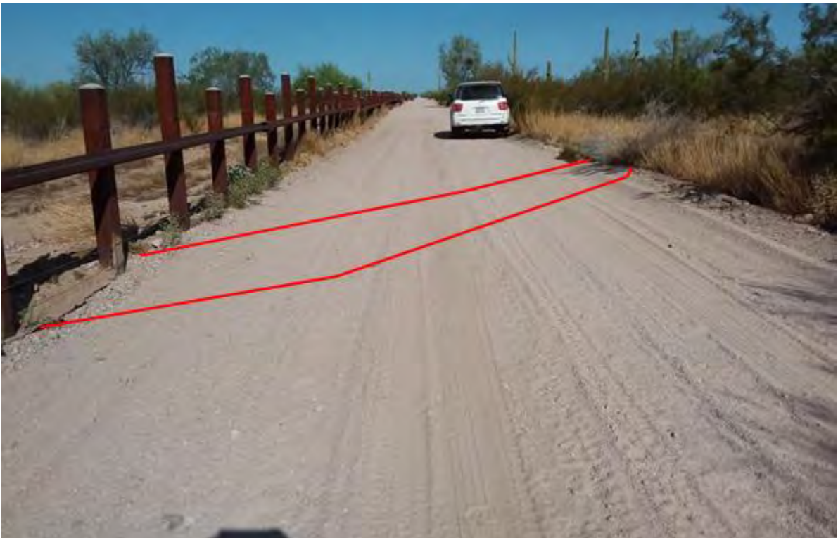
Figure 555. Photo point b11w1 looking west
