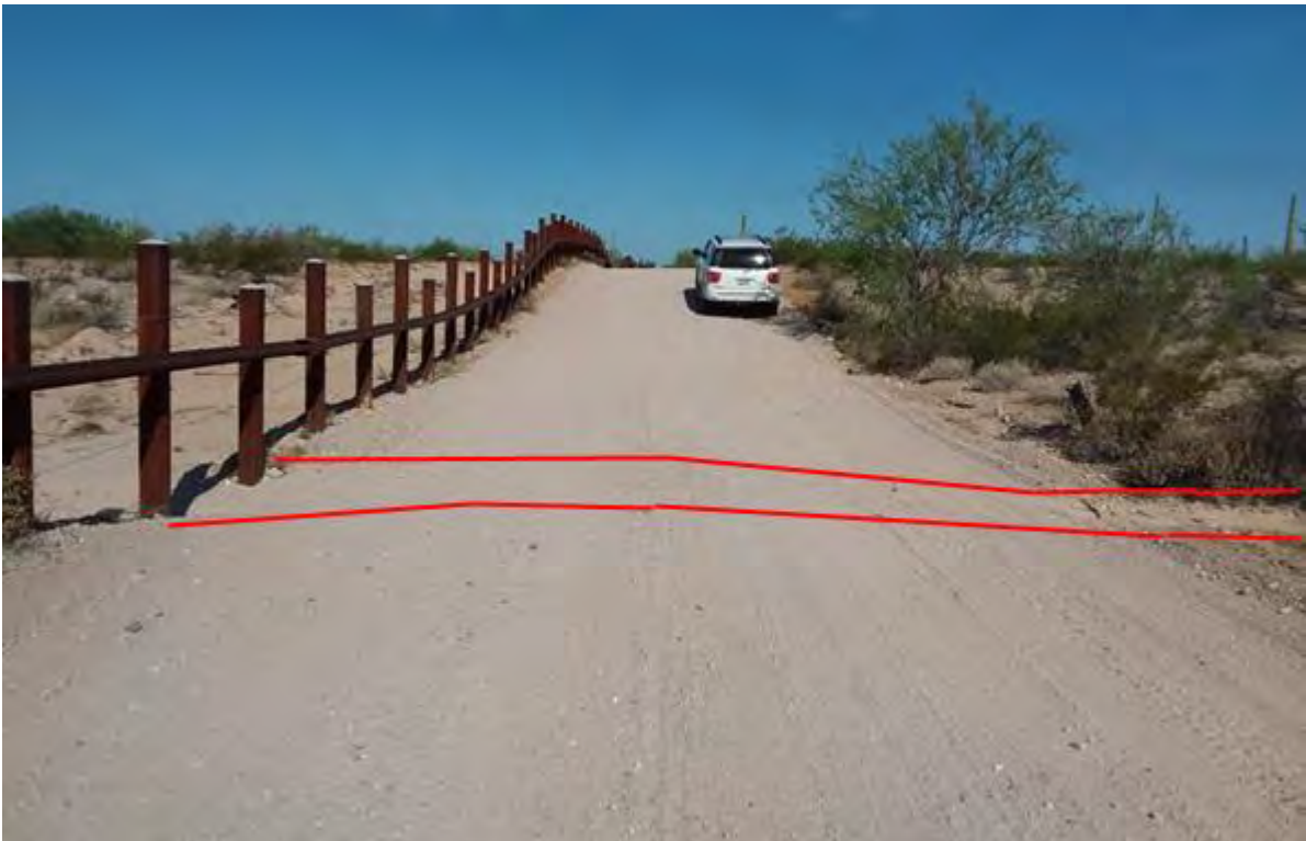
Figure 550. Photo point b10w1 looking west
