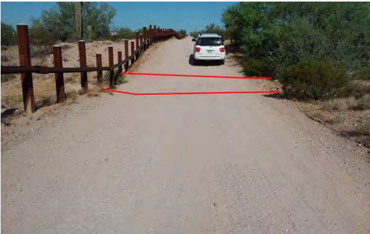
Figure 546. Photo point b10w3 looking west
