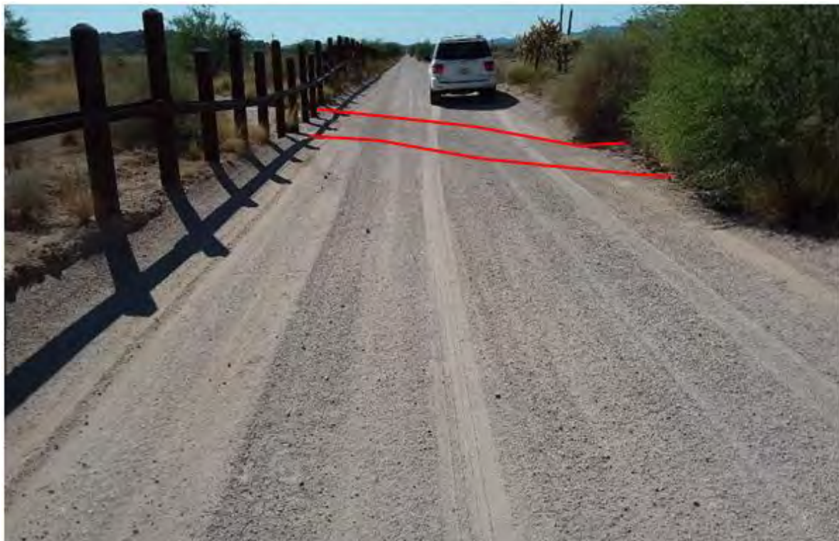
Figure 355. Photo point a35 looking upstream
