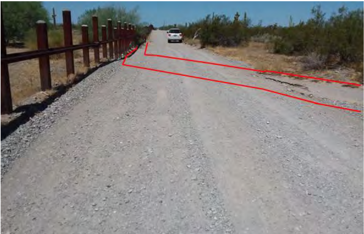
Figure 473. Photo point b8w1 looking west
