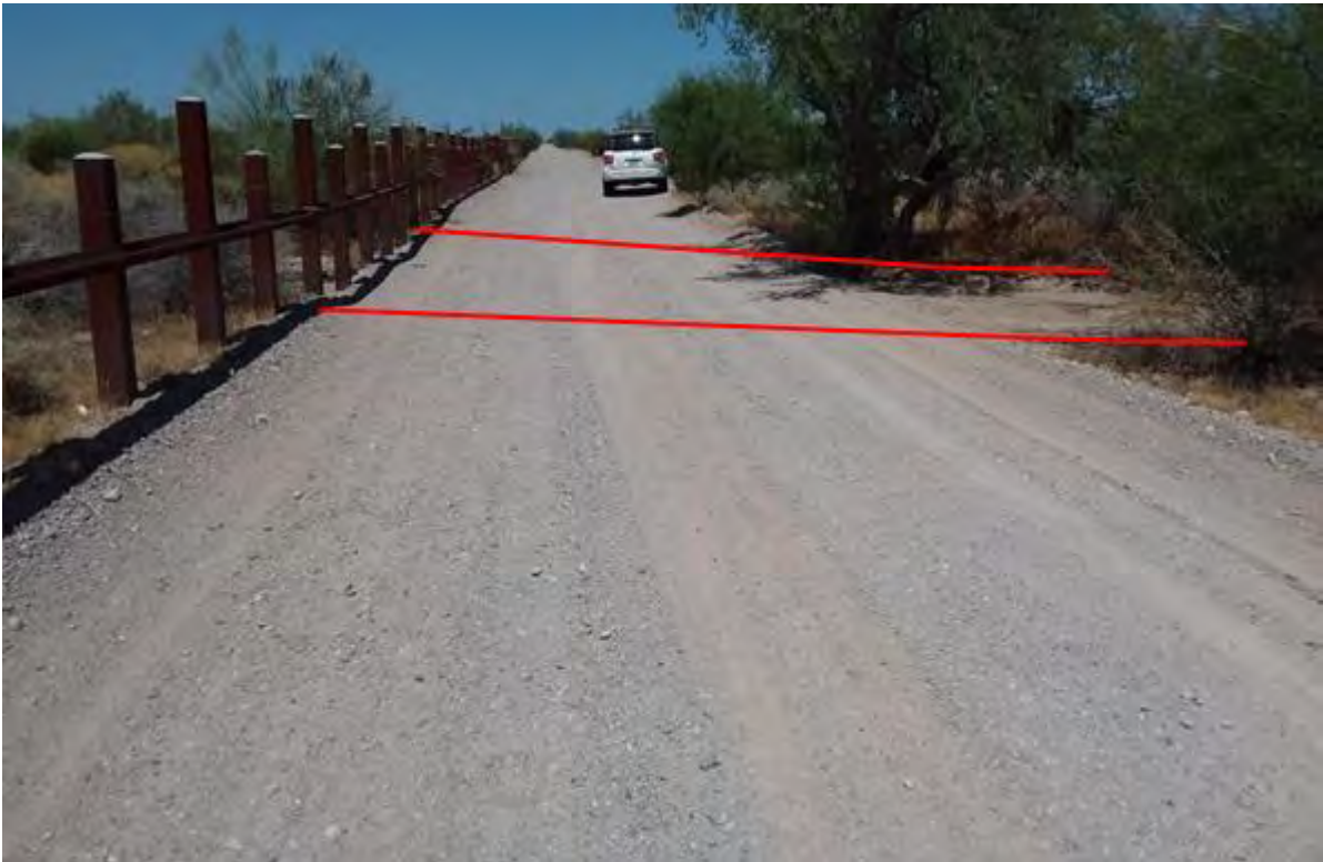
Figure 486. Photo point b9w13 looking west
