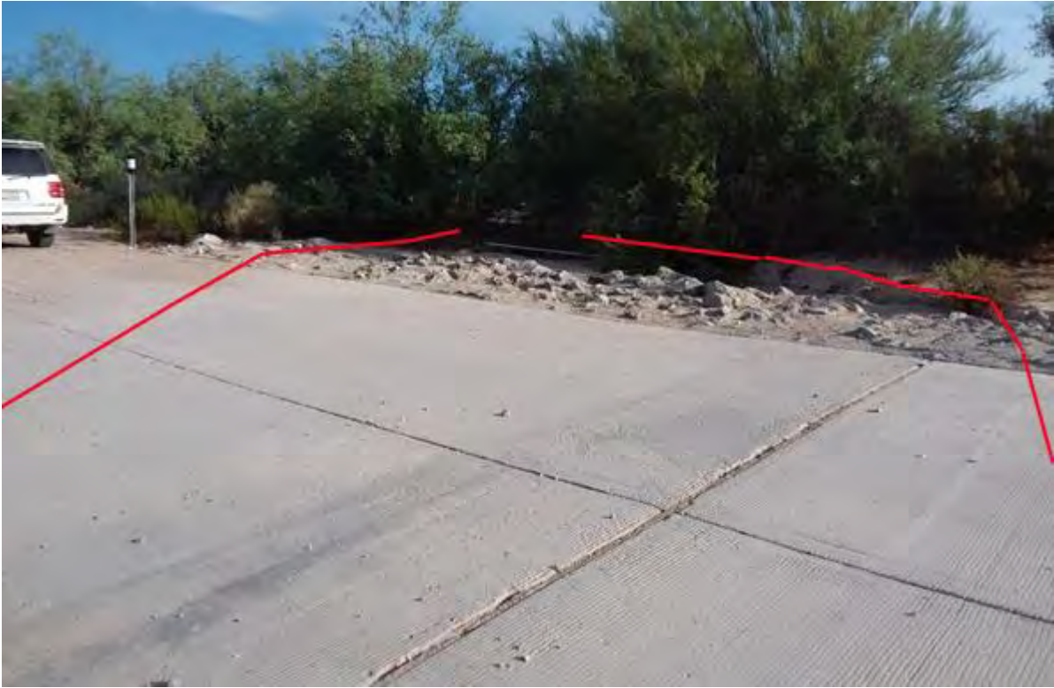
Figure 581. Photo point b13 looking upstream
