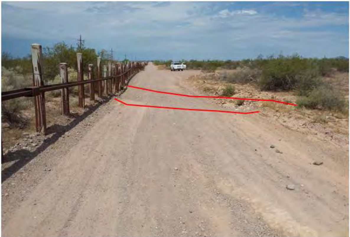
Figure 678. Photo point c2e6 looking west
