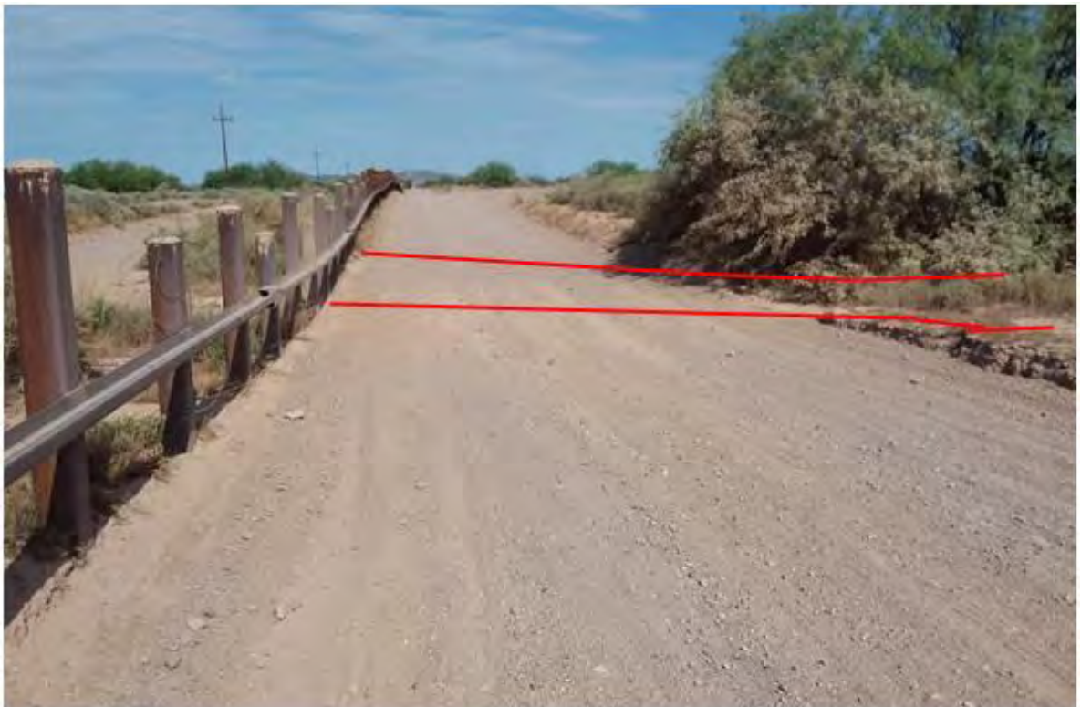
Figure 649. Photo point c0e3 looking west
