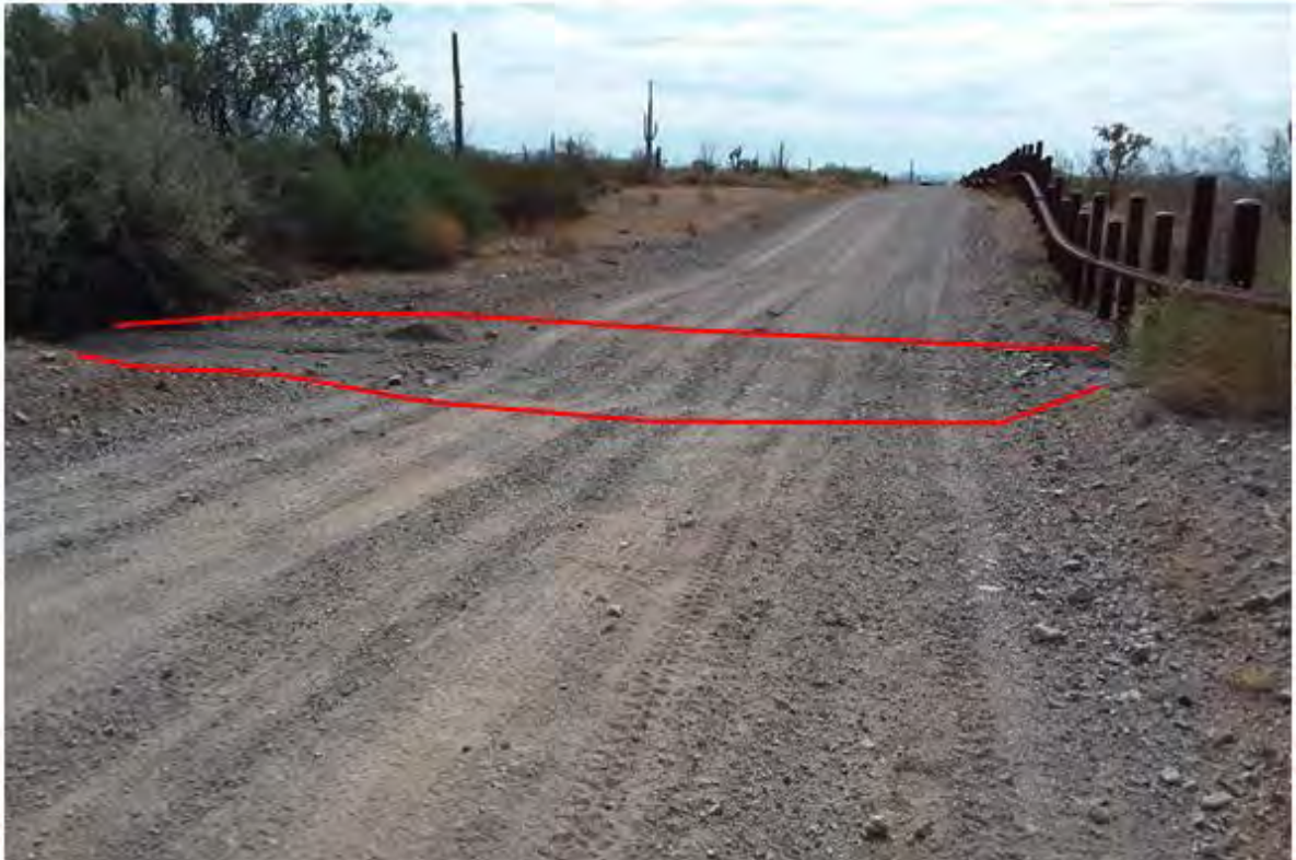
Figure 238. Photo point a17 looking east
