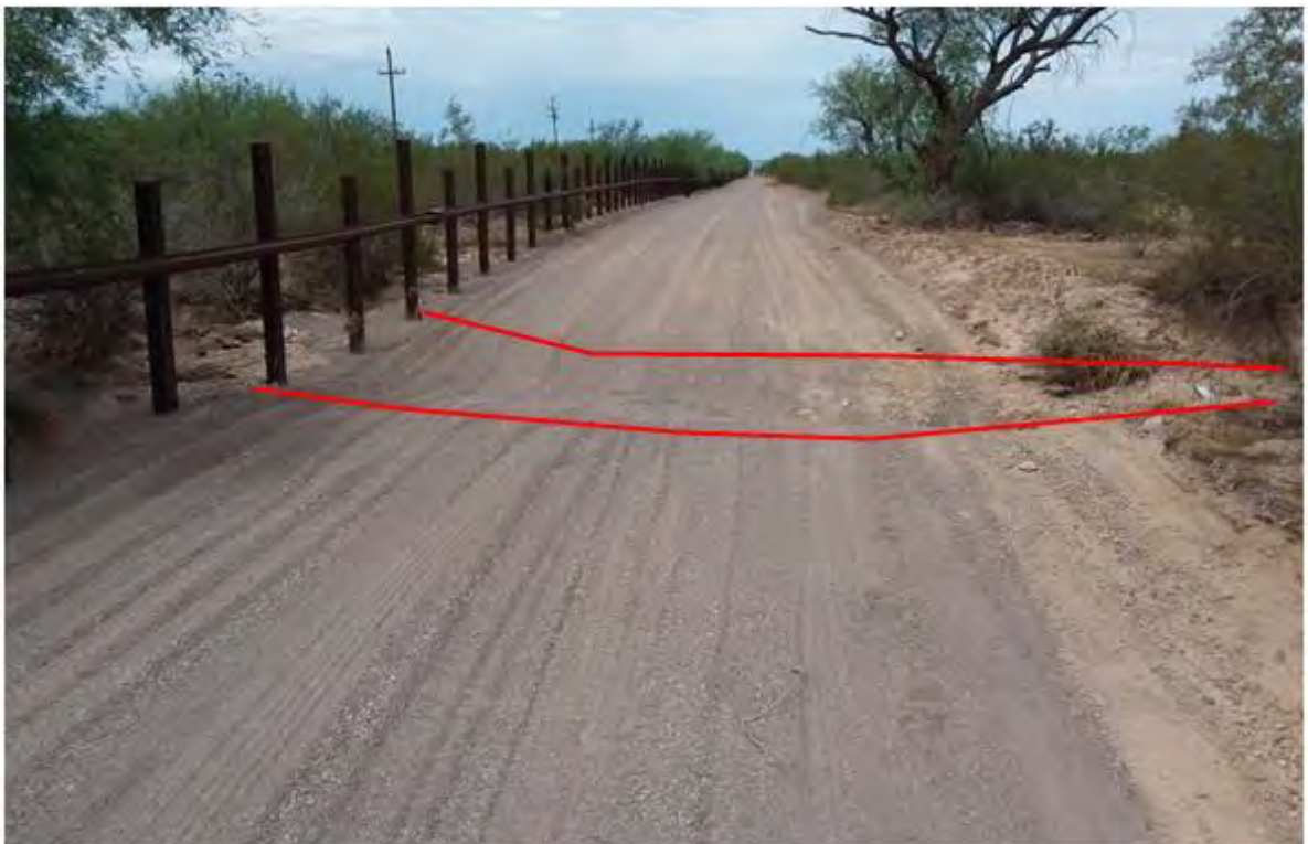
Figure 696. Photo point c4e2 looking west
