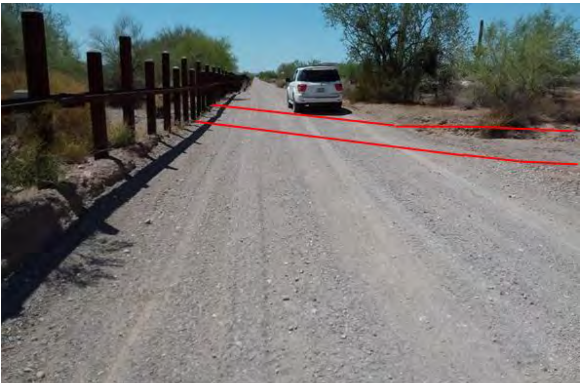
Figure 404. Photo point b3w6 looking west
