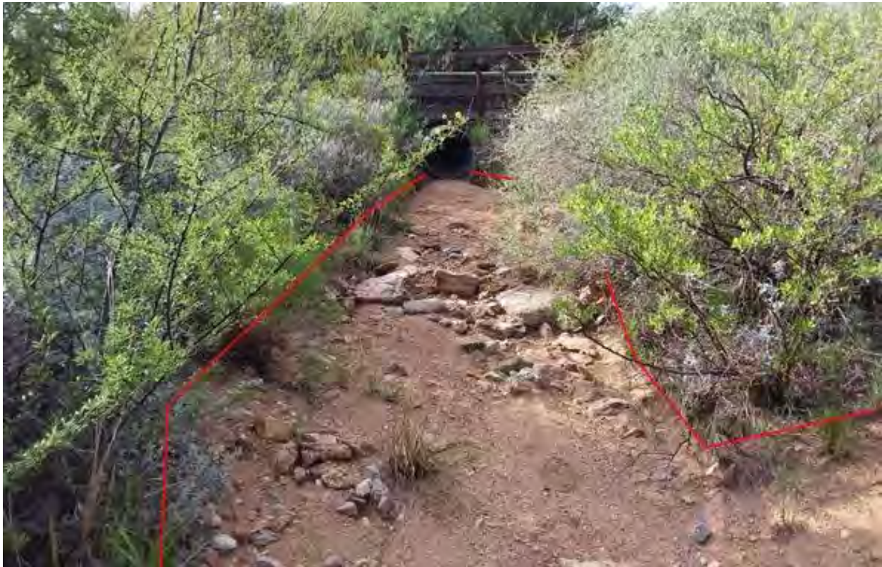
Figure 817. Photo point a4 looking upstream
