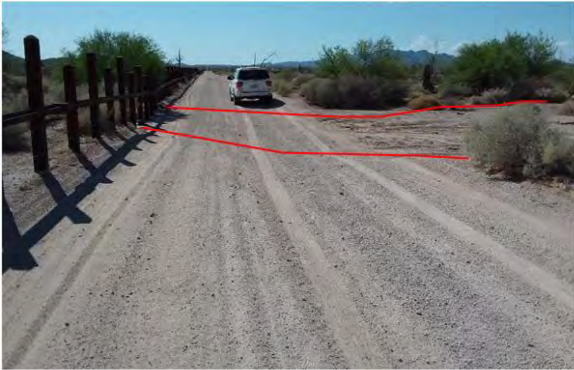
Figure 357. Photo point b1w7 looking west
