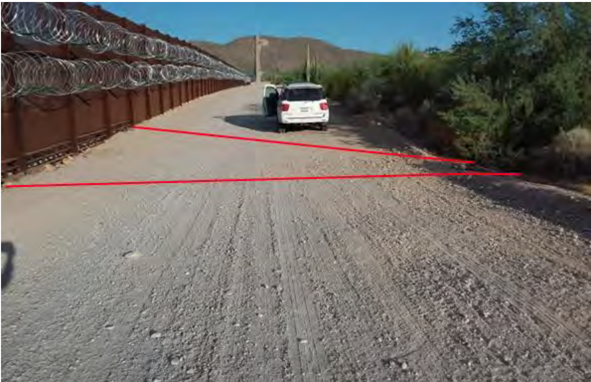
Figure 588. Photo point b15w4 looking west
