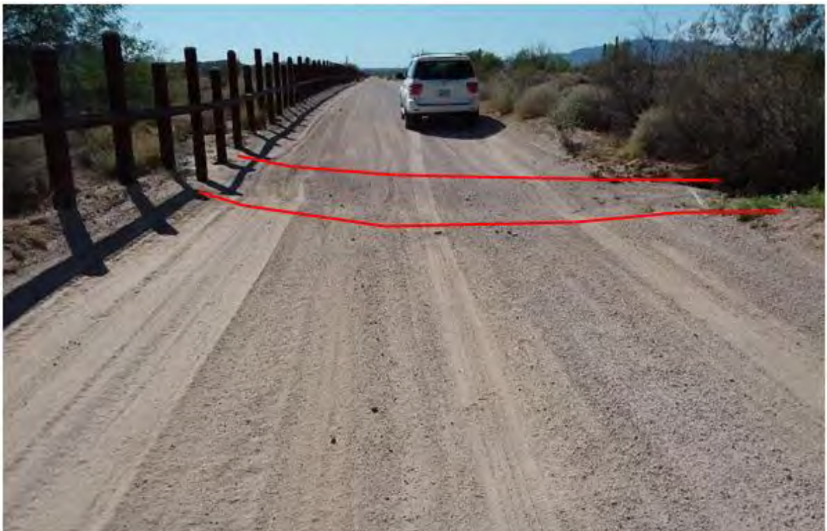
Figure 360. Photo point b1w6 looking west
