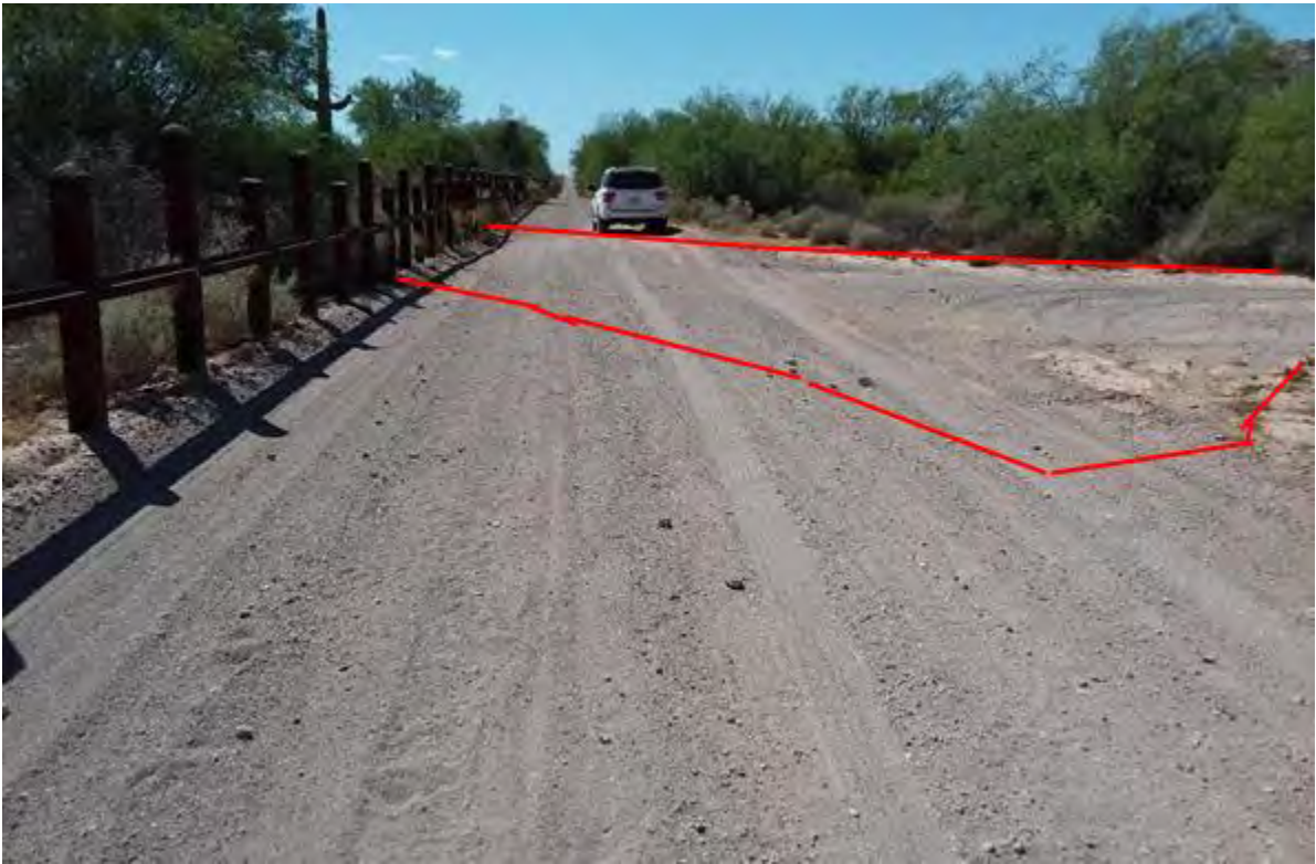
Figure 380. Photo point b2w1 looking west
