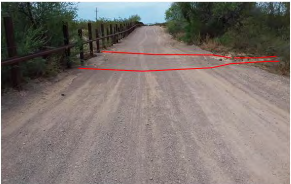
Figure 701. Photo point c4e4 looking west
