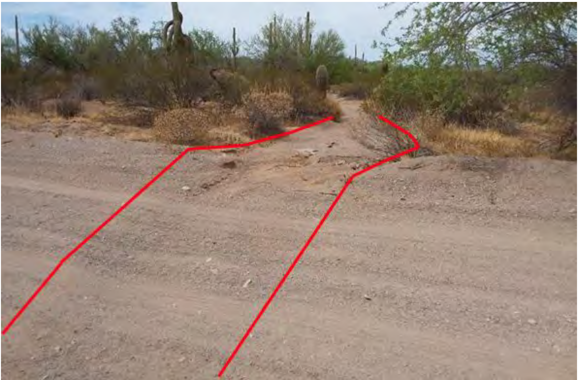
Figure 47. Photo point a5 looking upstream
