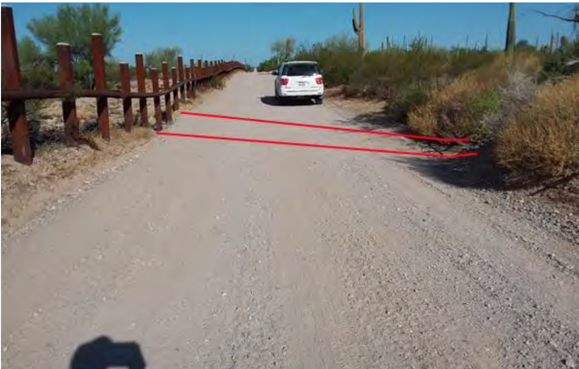
Figure 562. Photo point b13w8 looking west
