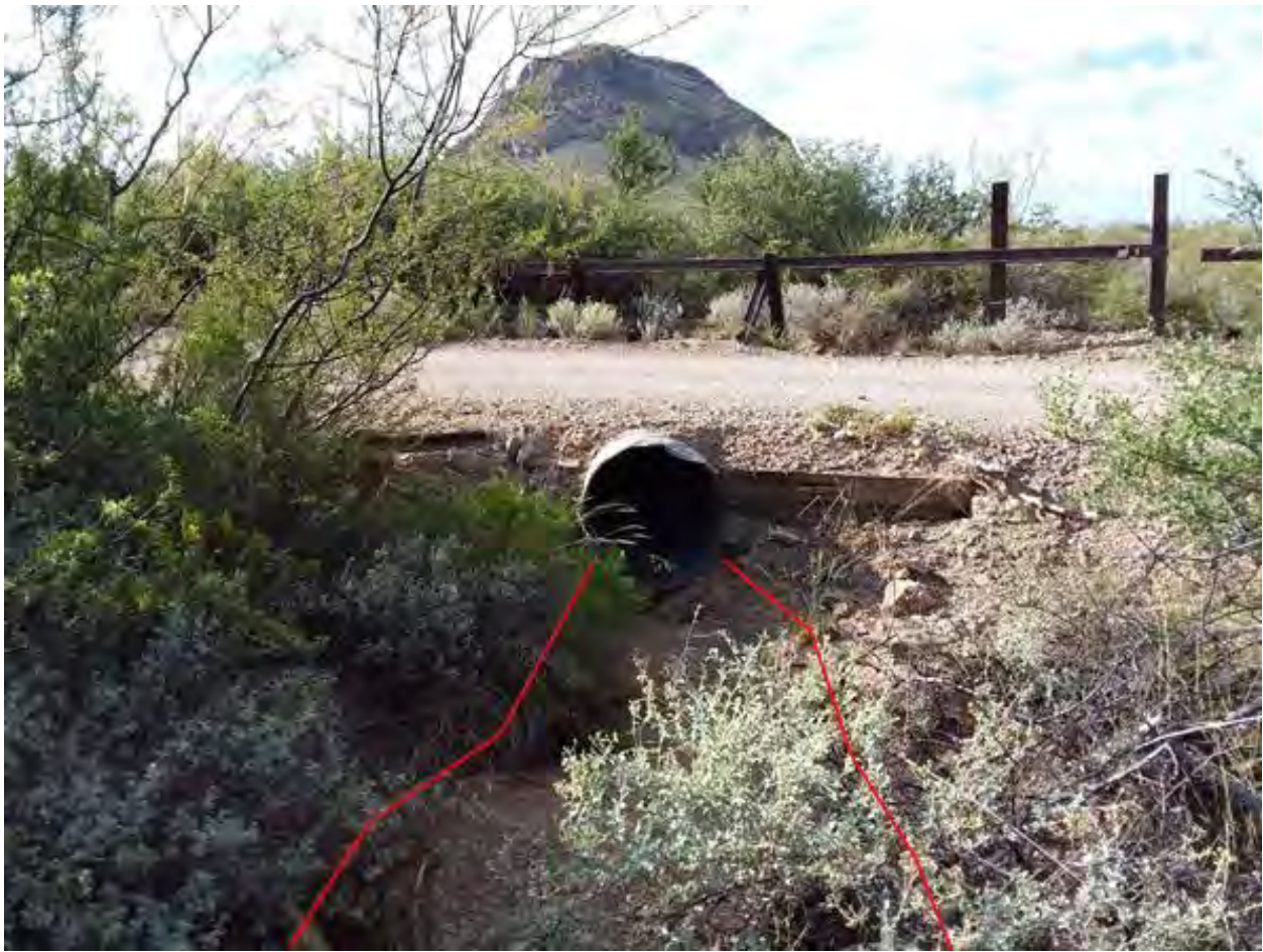
Figure 819. Photo point a5 looking upstream towards culvert
