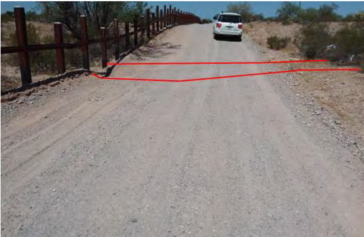
Figure 489. Photo point b9w12 looking west
