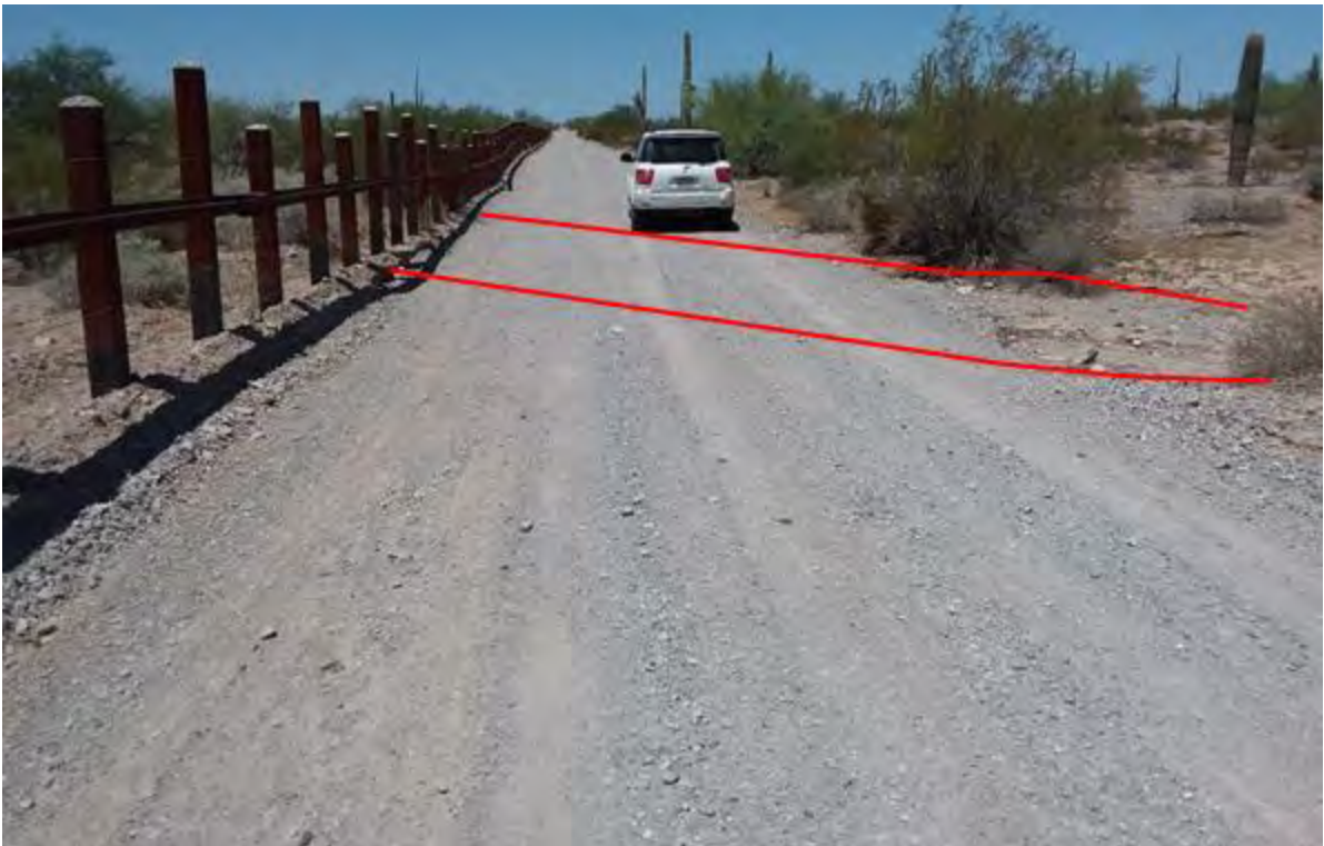
Figure 454. Photo point b6w1 looking west
