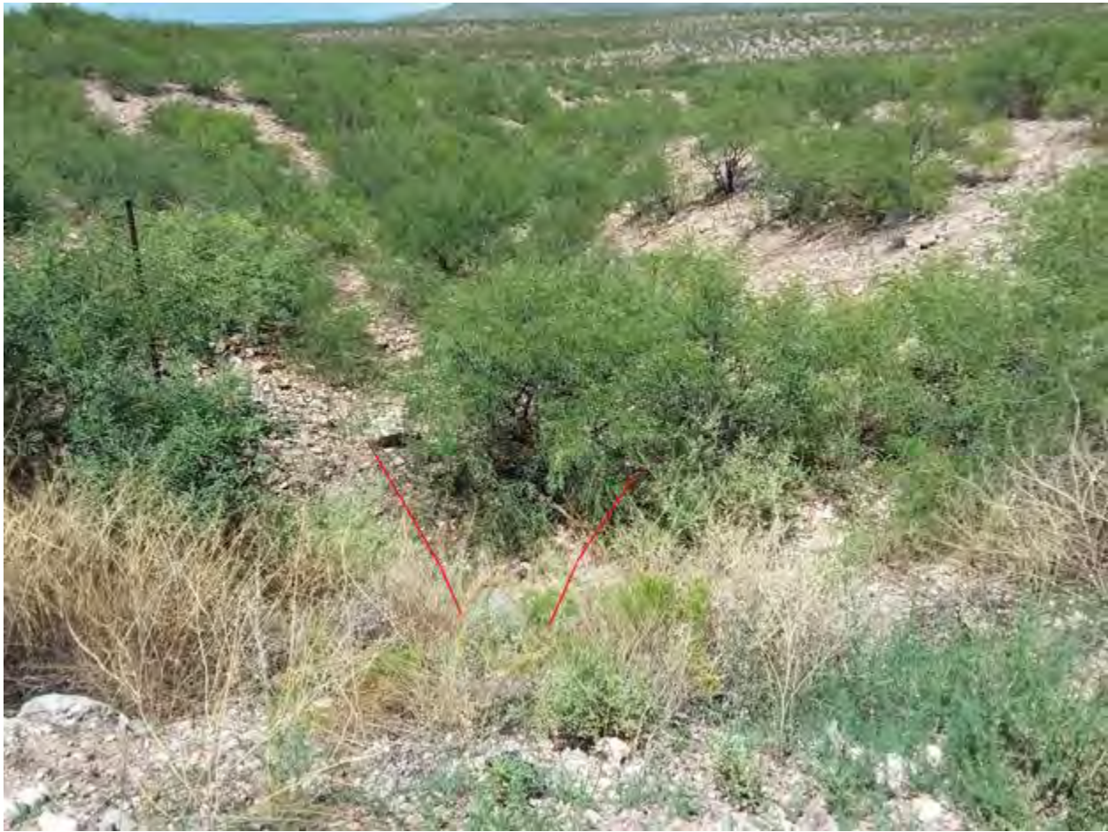
Figure 920. Photo point e16 looking downstream at culvert outlet
