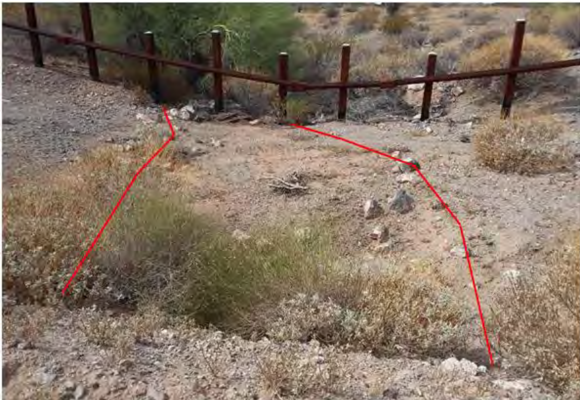
Figure 231. Photo point a17w3 looking downstream from culverts Double culverts under road
