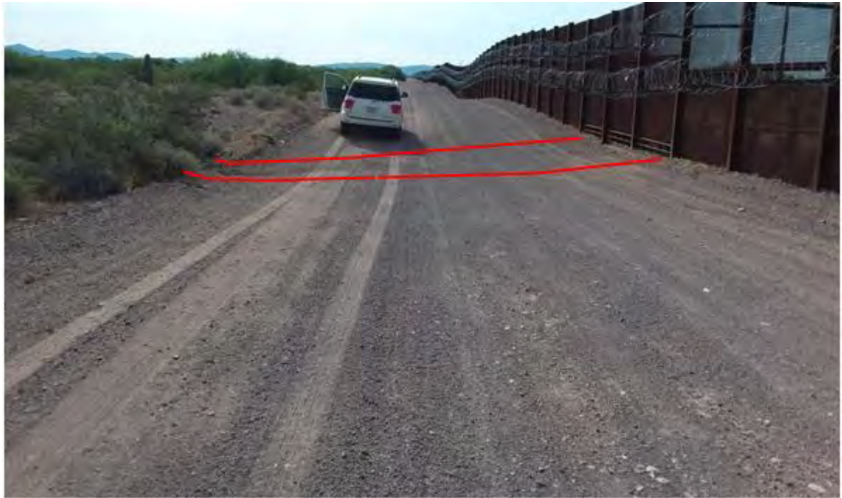
Figure 630. Photo point b18e6 looking east
