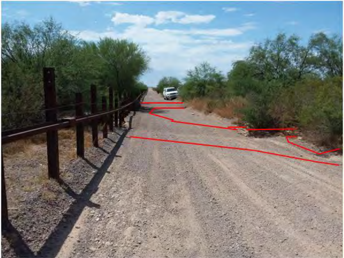
Figure 736. Photo point c5e1 looking west
