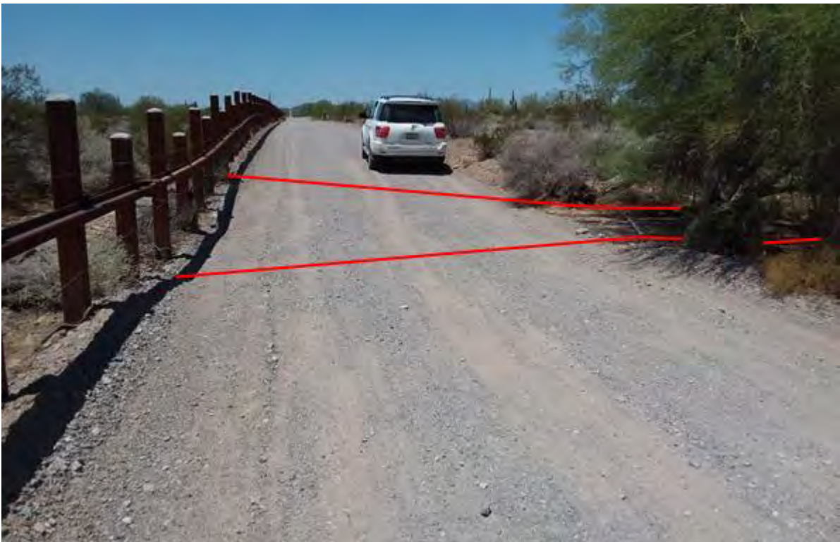
Figure 444. Photo point b5w1 looking west
