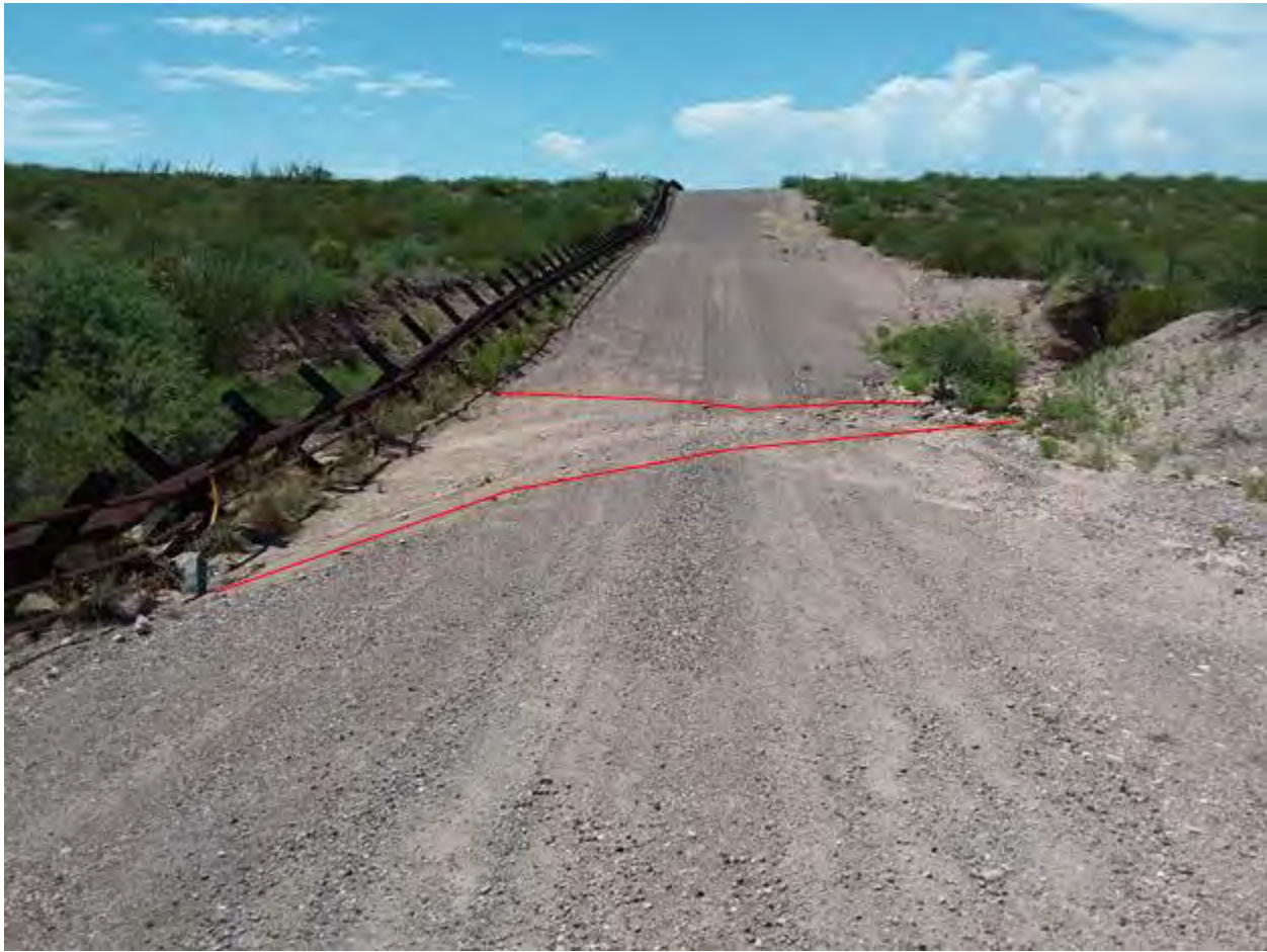
Figure 916. Photo point e14 looking west
