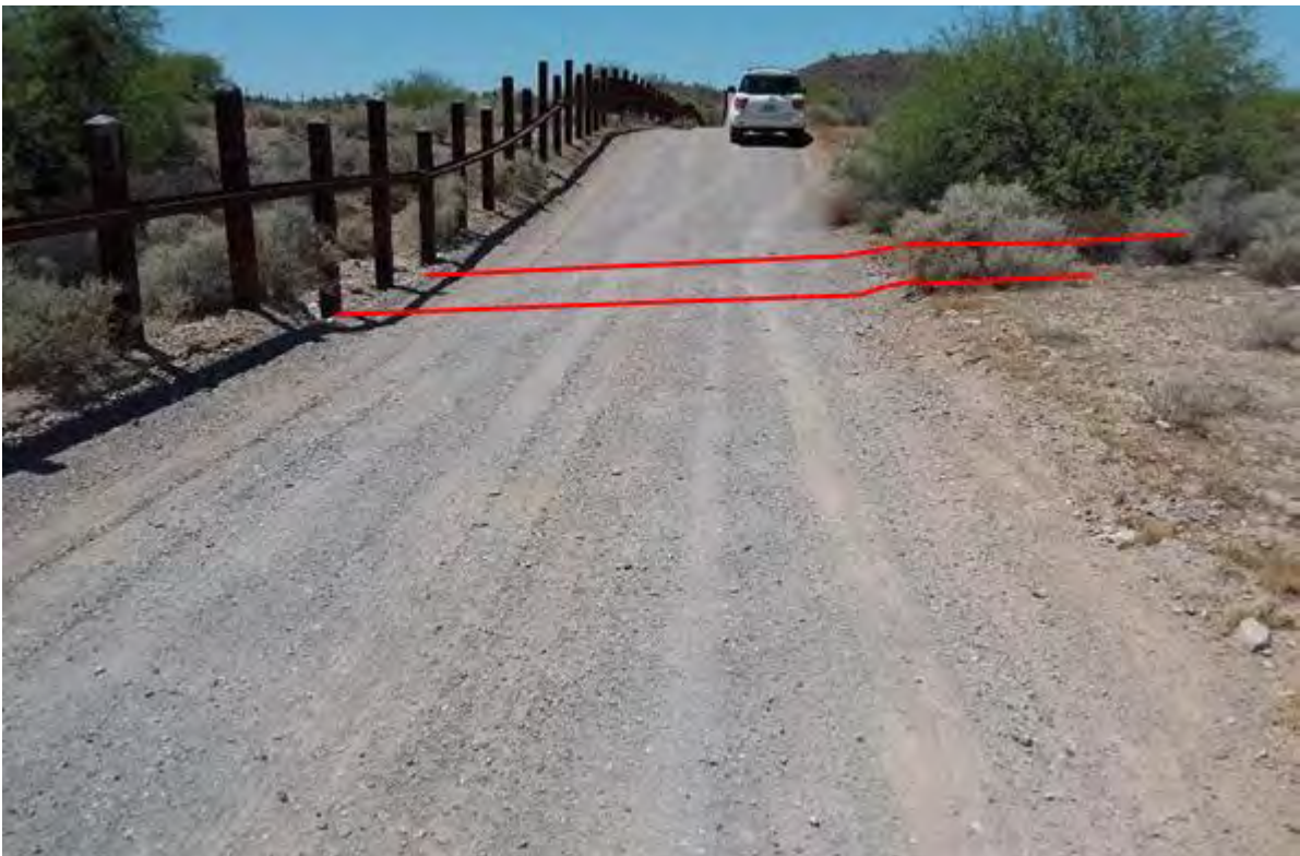
Figure 424. Photo point b4w2 looking west
