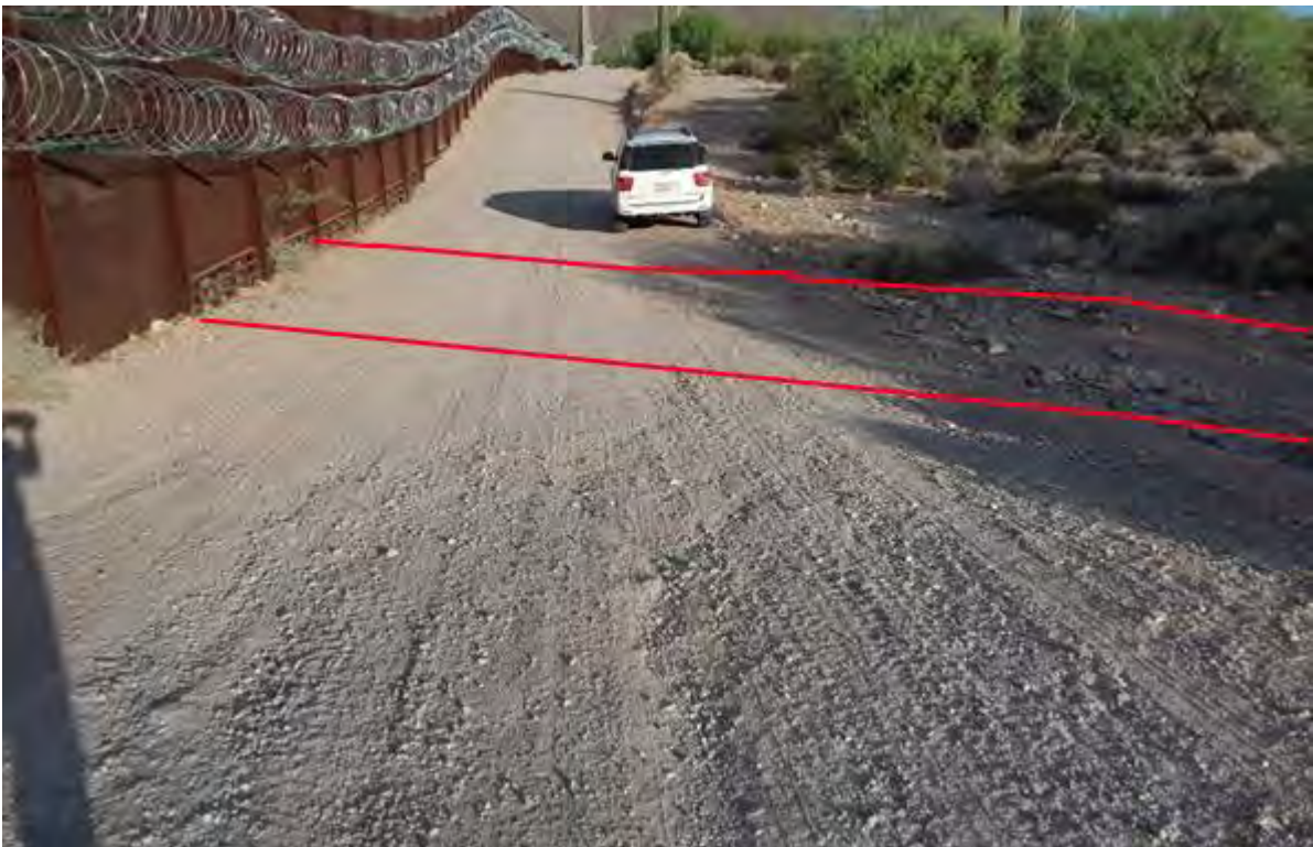
Figure 590. Photo point b15w3 looking west
