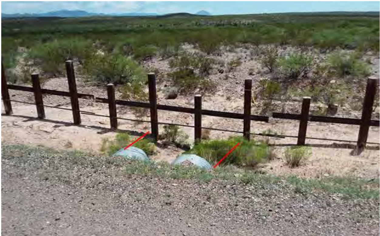
Figure 904. Photo point e8a looking downstream at culvert outlet
