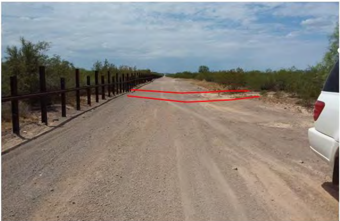
Figure 719. Photo point c4e11 looking west
