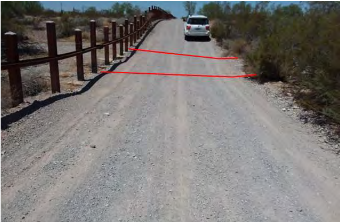
Figure 449. Photo point b6w3 looking west
