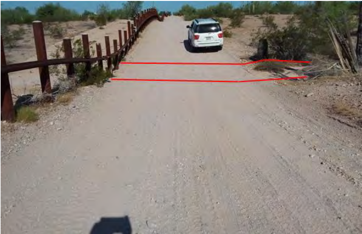
Figure 548. Photo point b10w2 looking west
