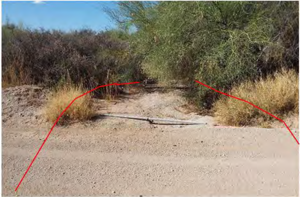
Figure 339. Photo point a34b looking upstream
