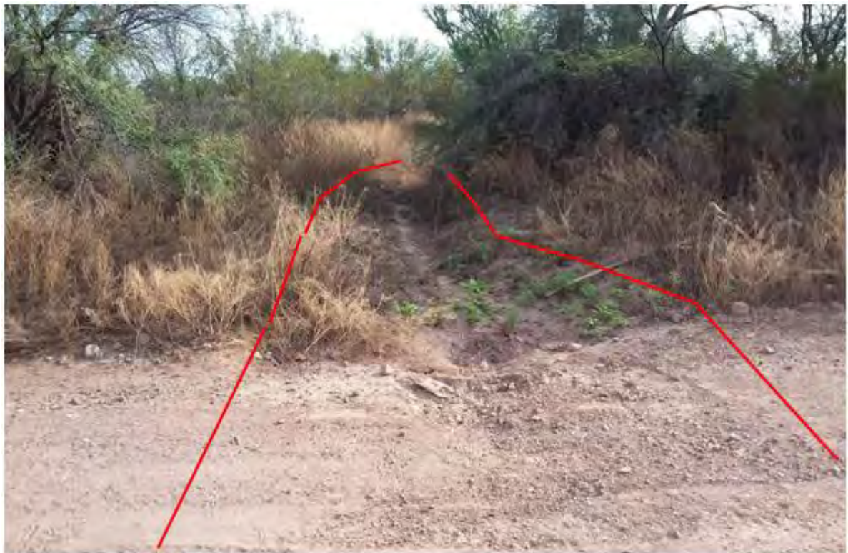
Figure 620. Photo point b18e1 looking upstream
