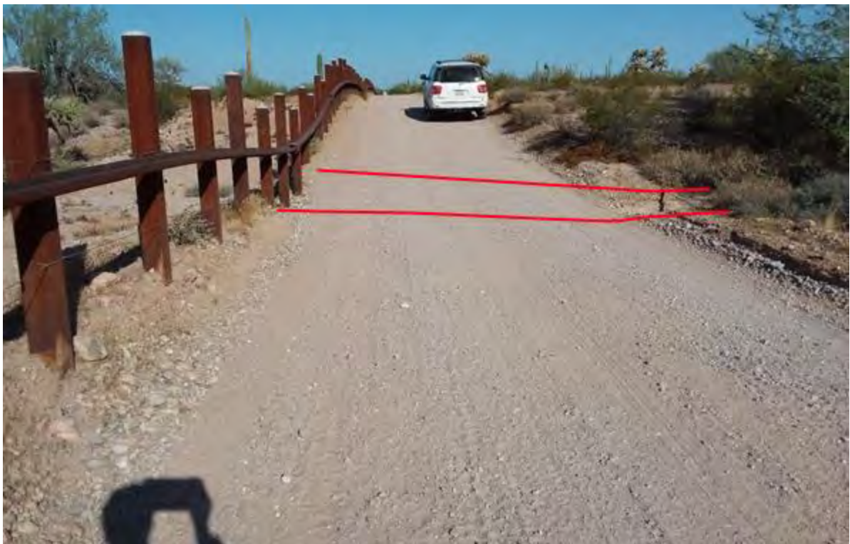
Figure 565. Photo point b13w7 looking west
