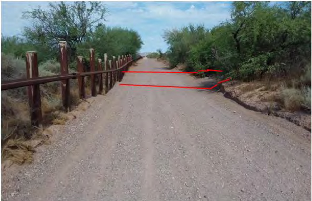
Figure 655. Photo point c0e5 looking west
