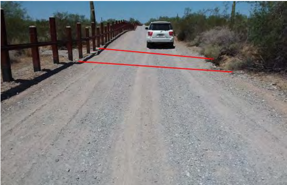
Figure 461. Photo point b7w1 looking west
