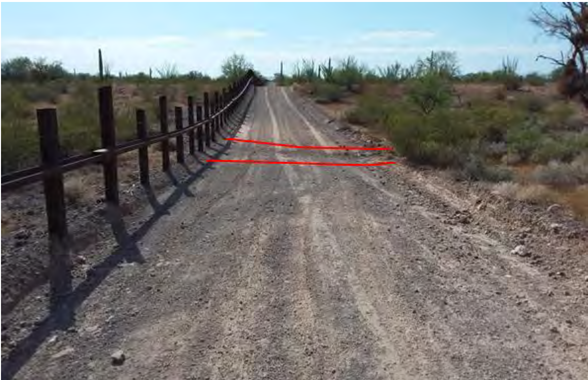
Figure 779. Photo point c7e3 looking west
