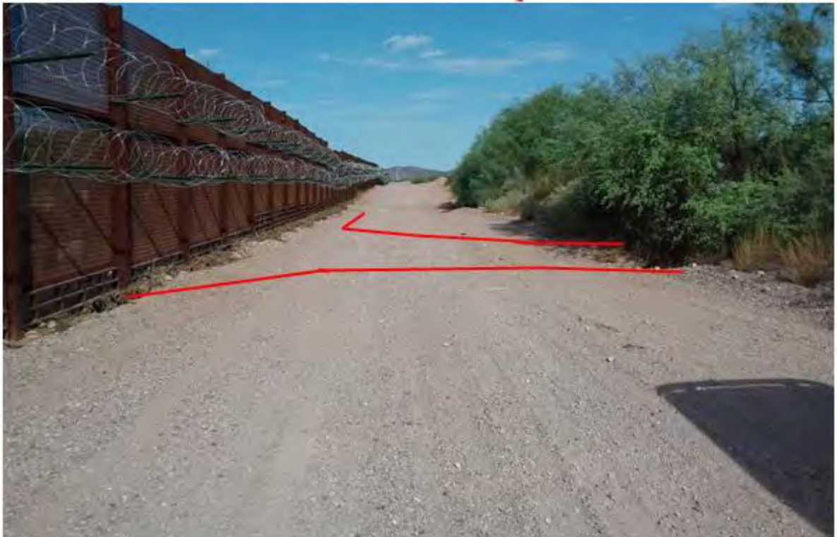
Figure 638. Photo point b18e9 looking west
