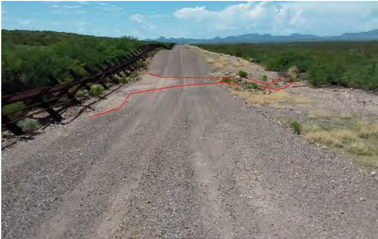
Figure 914. Photo point e13 looking west
