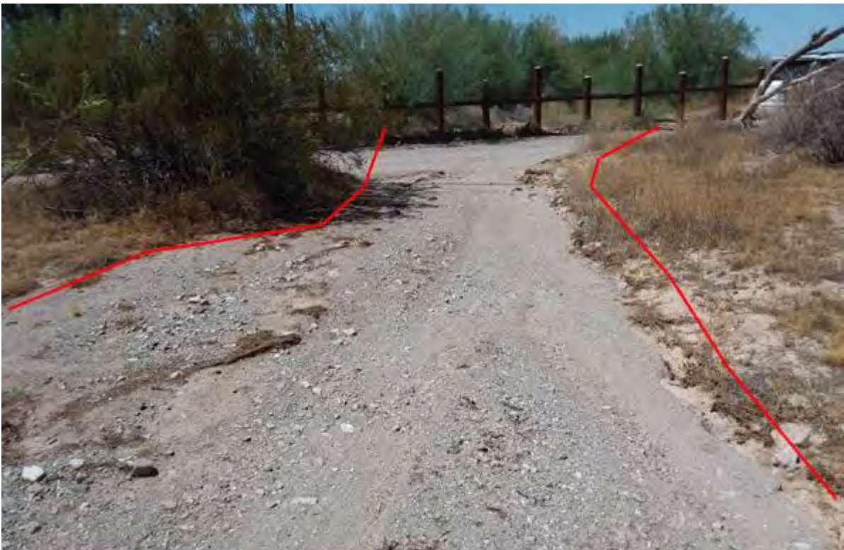
Figure 471. Photo point b8w1b looking downstream
