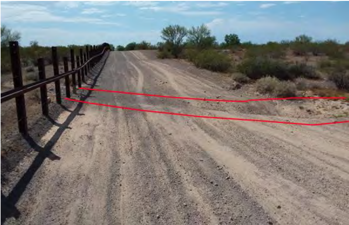
Figure 754. Photo point c6e2 looking west
