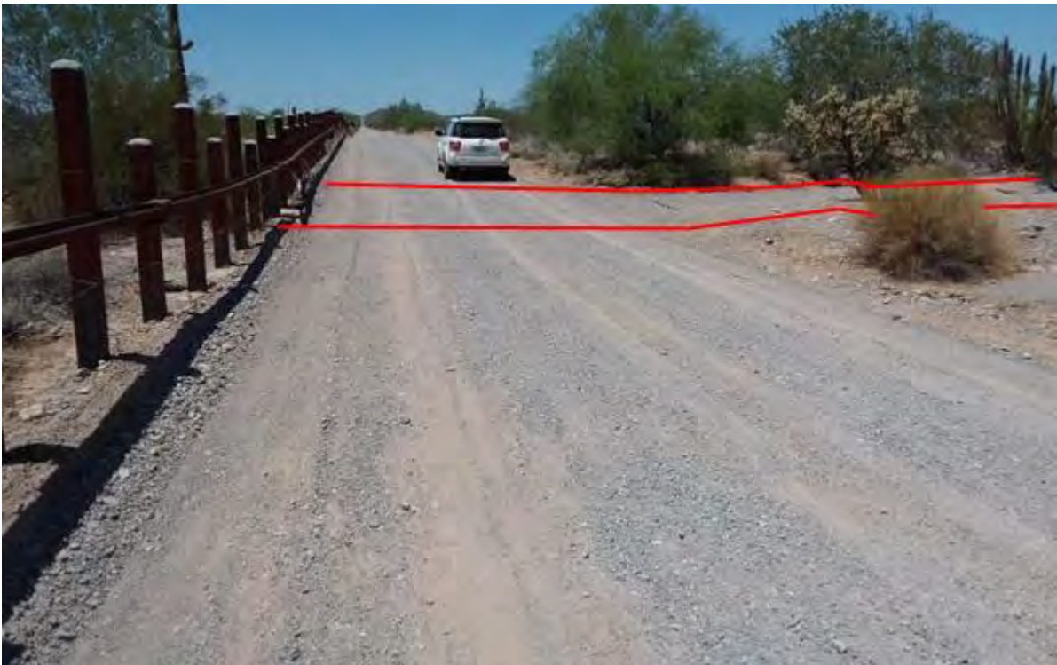
Figure 441. Photo point b5w2 looking west
