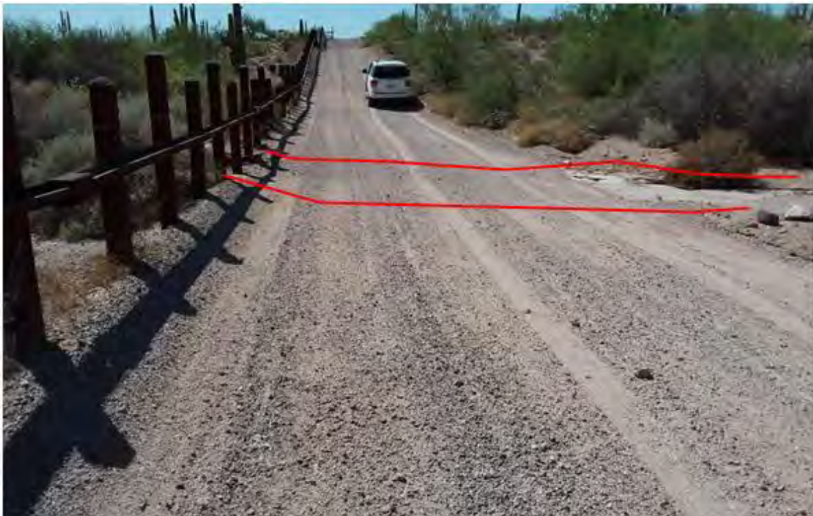
Figure 374. Photo point b1w1 looking west
