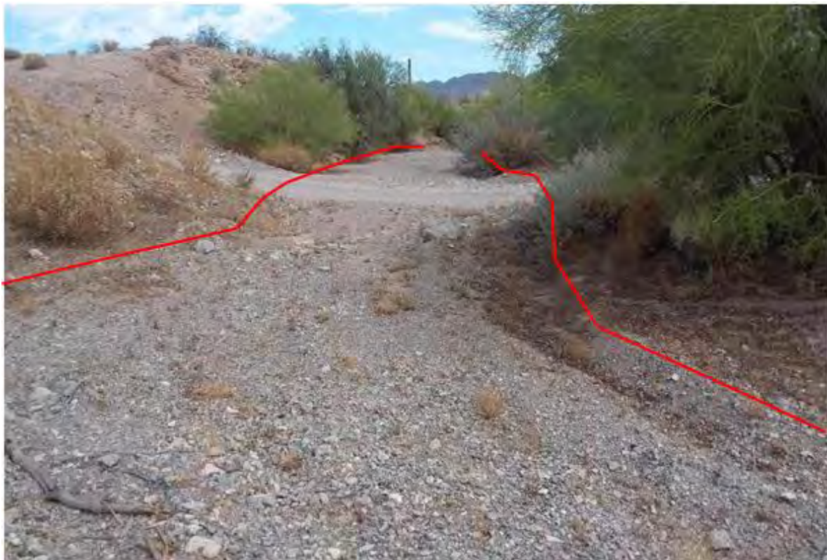
Figure 219. Photo point a16 looking upstream
