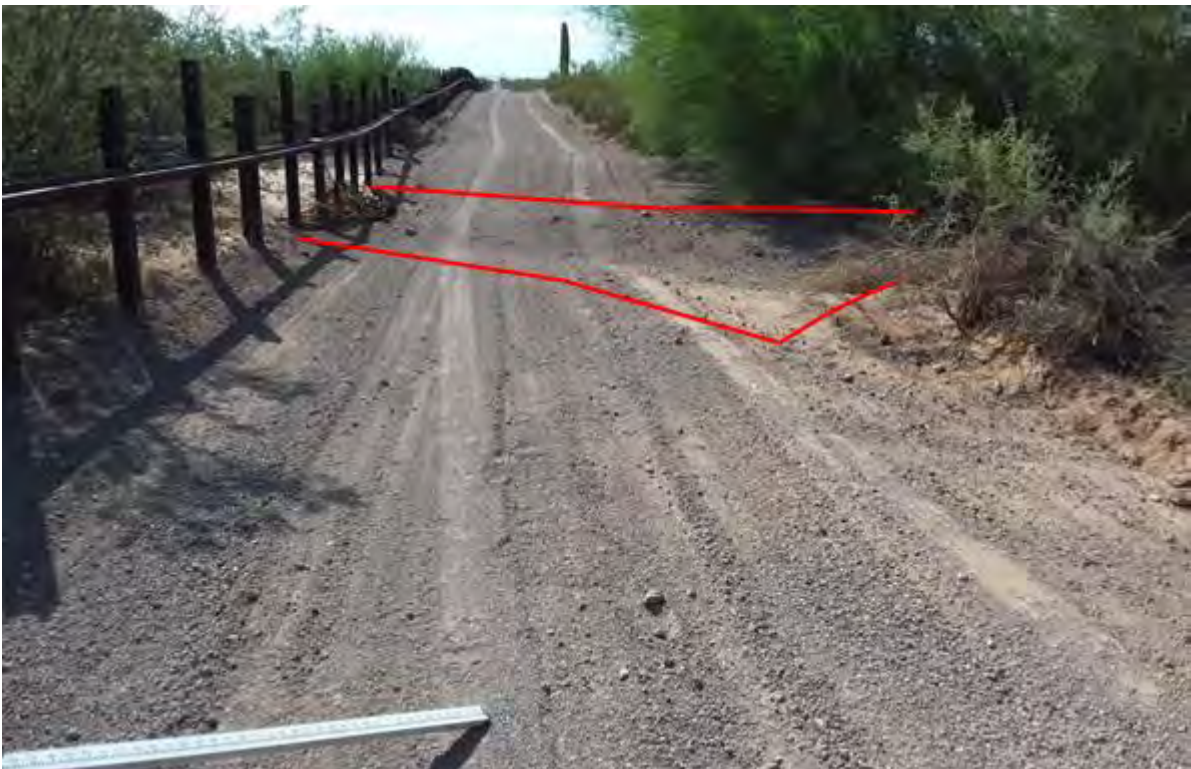
Figure 774. Photo point c7e1 looking west
