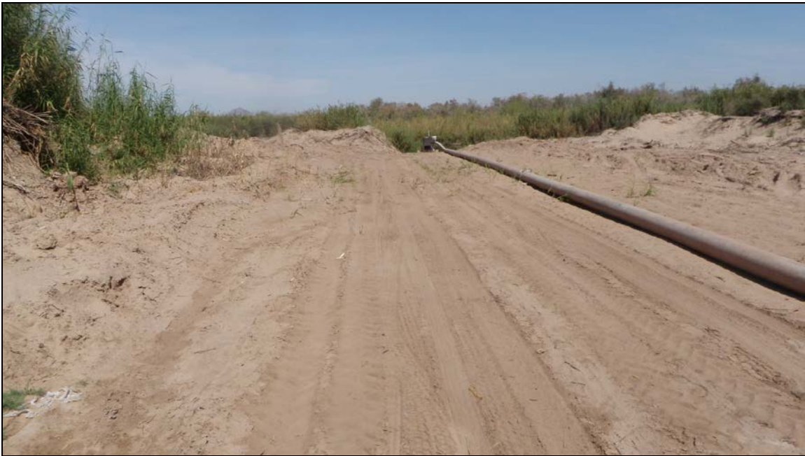
PHOTOGRAPH 5: Central grubbed area across jurisdictional wetlands. Two water pumps and 12-inch-diameter water pipe were observed.
