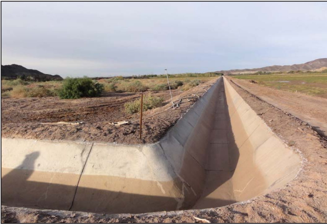
PHOTOGRAPH 3 Proposed Irrigation Channel; Tie-in Location
