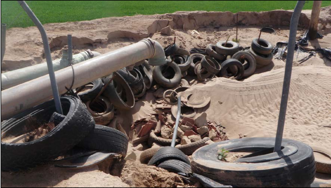
PHOTOGRAPH 8: Detail of spigot at southern terminus of water pipe in central grubbed area.
