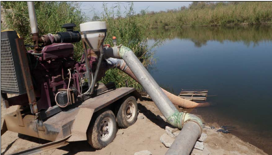
PHOTOGRAPH 7: Detail of pump drawing water from main channel of the Colorado River in central grubbed area.
