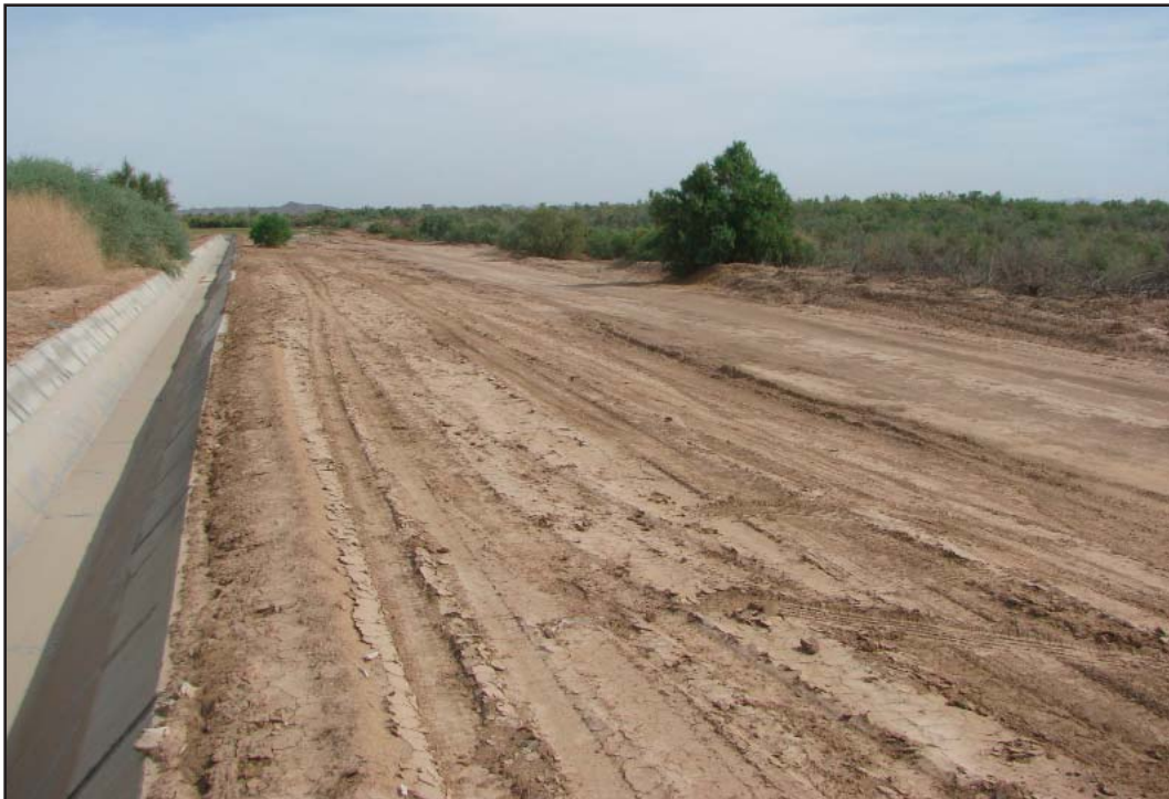
PHOTOGRAPH 8 Western Maintenance Access Road
