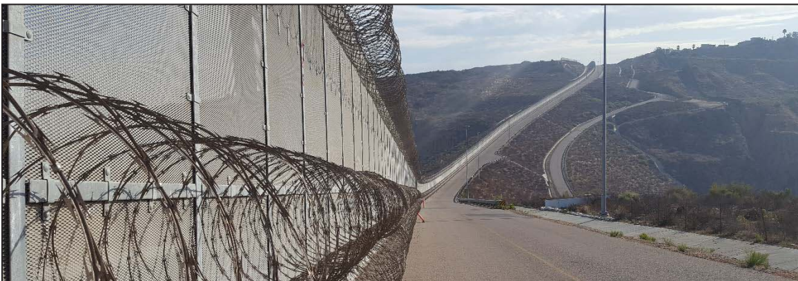
Photograph 5.3 Secondary Fence and existing all-weather road in the Western Segment. Primary Fence is delineated to the right.
