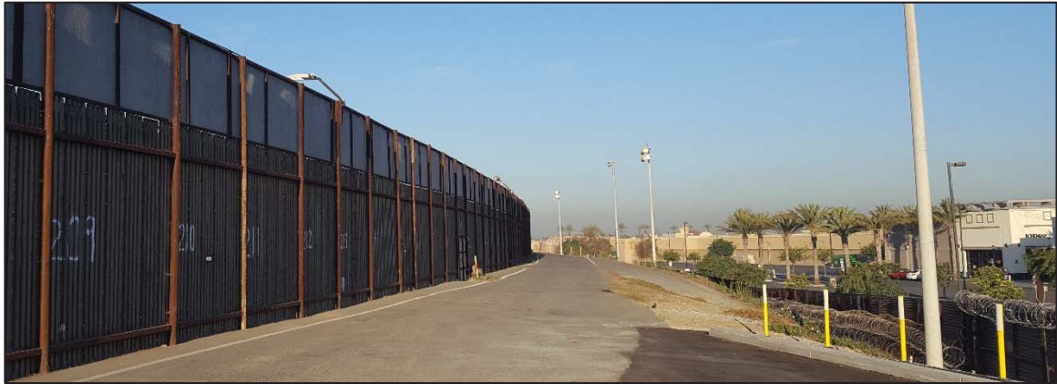
Photograph 5.4 Northern Levee Segment: The fence on the left parallels the Tijuana River Floodway and will be replaced with the new Primary Fence for a distance of approximately 1,200 feet.
