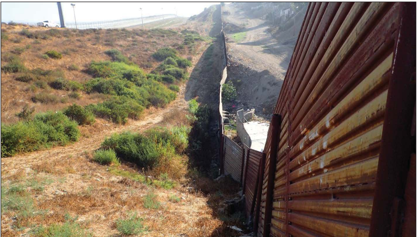
Photograph 2.2 Existing Primary Fence. View of extent of existing primary fence in the Project Area.
