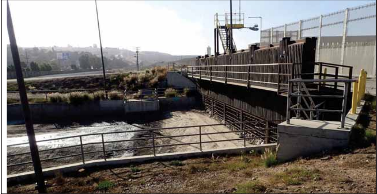
Photograph 15. Example of a non-jurisdictional concrete drainage, located to the southeast of the waste treatment facility. View facing west. Photograph taken on October 13, 2017.
