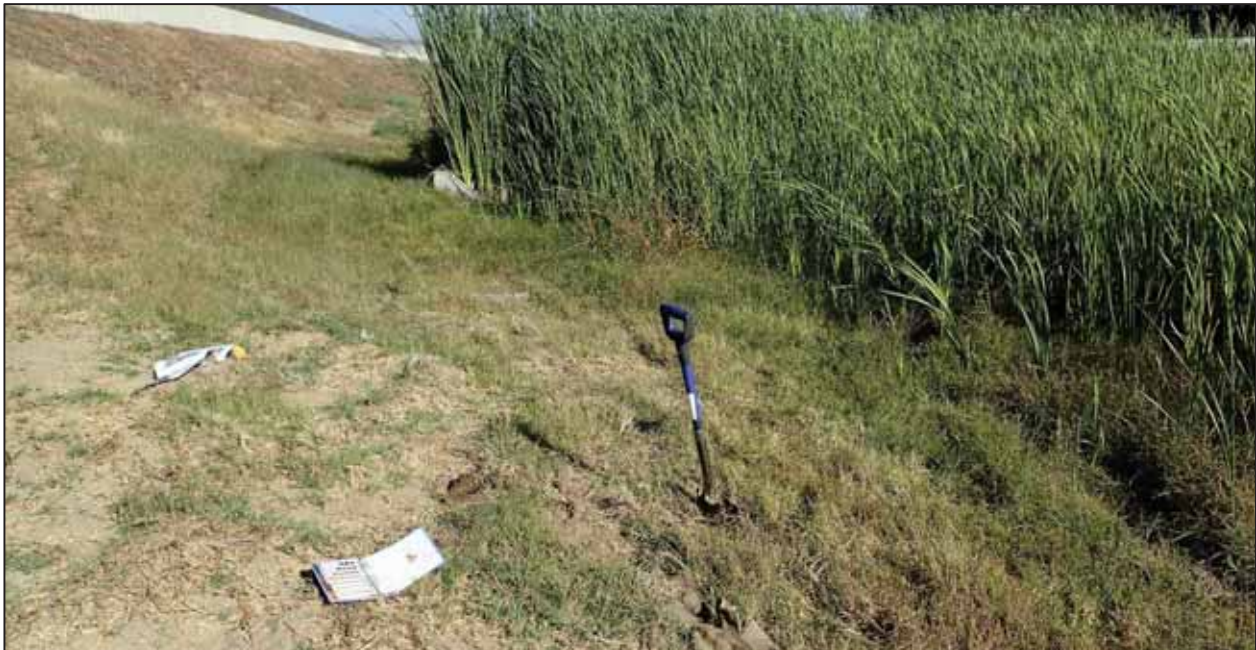
Photograph 2. Emergent marsh, W02, a saturated and inundated area at the entrance to a culvert, south of the water treatment plant west of the Tijuana River. The feature is dominated by cattails and barnyard grass. View facing east. Photograph taken on October 10, 2017.
