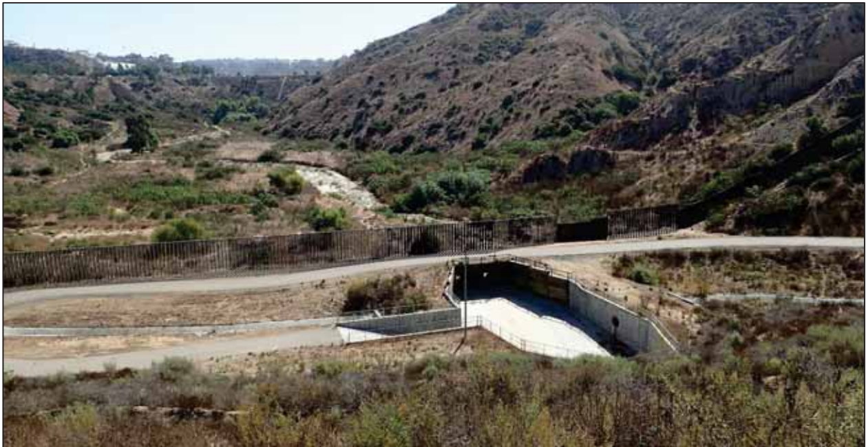
Photograph 12. Image depicts S07, the natural and concrete channelized portion of the ephemeral drainage in Smugglers Gulch. View facing south. Photograph taken October 10, 2017.
