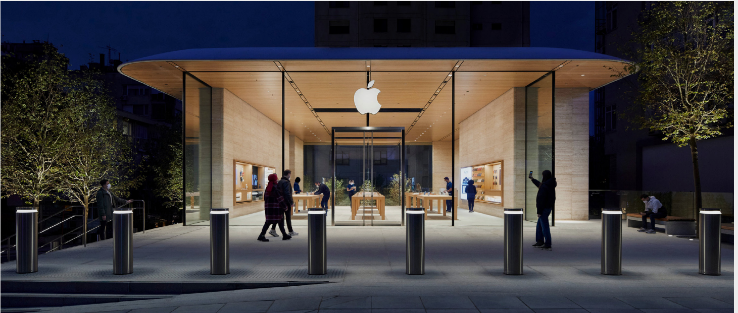
In 2021, we opened Apple Bağdat Caddesi with environmental features, including natural lighting and rainwater capture.
