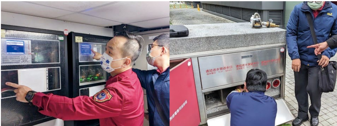
Fire Agencies Conducted Fire Safety Equipment Inspections
