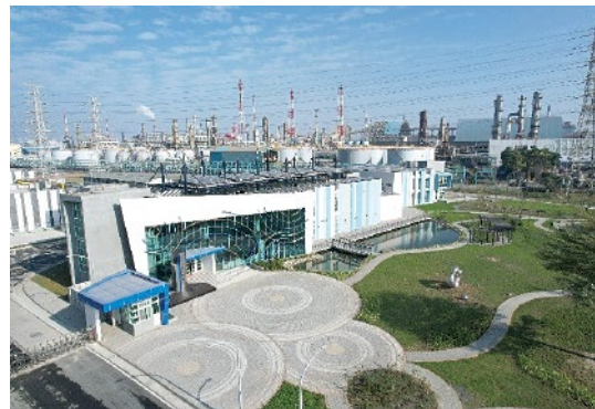
Linhai Water Reclamation Plant
