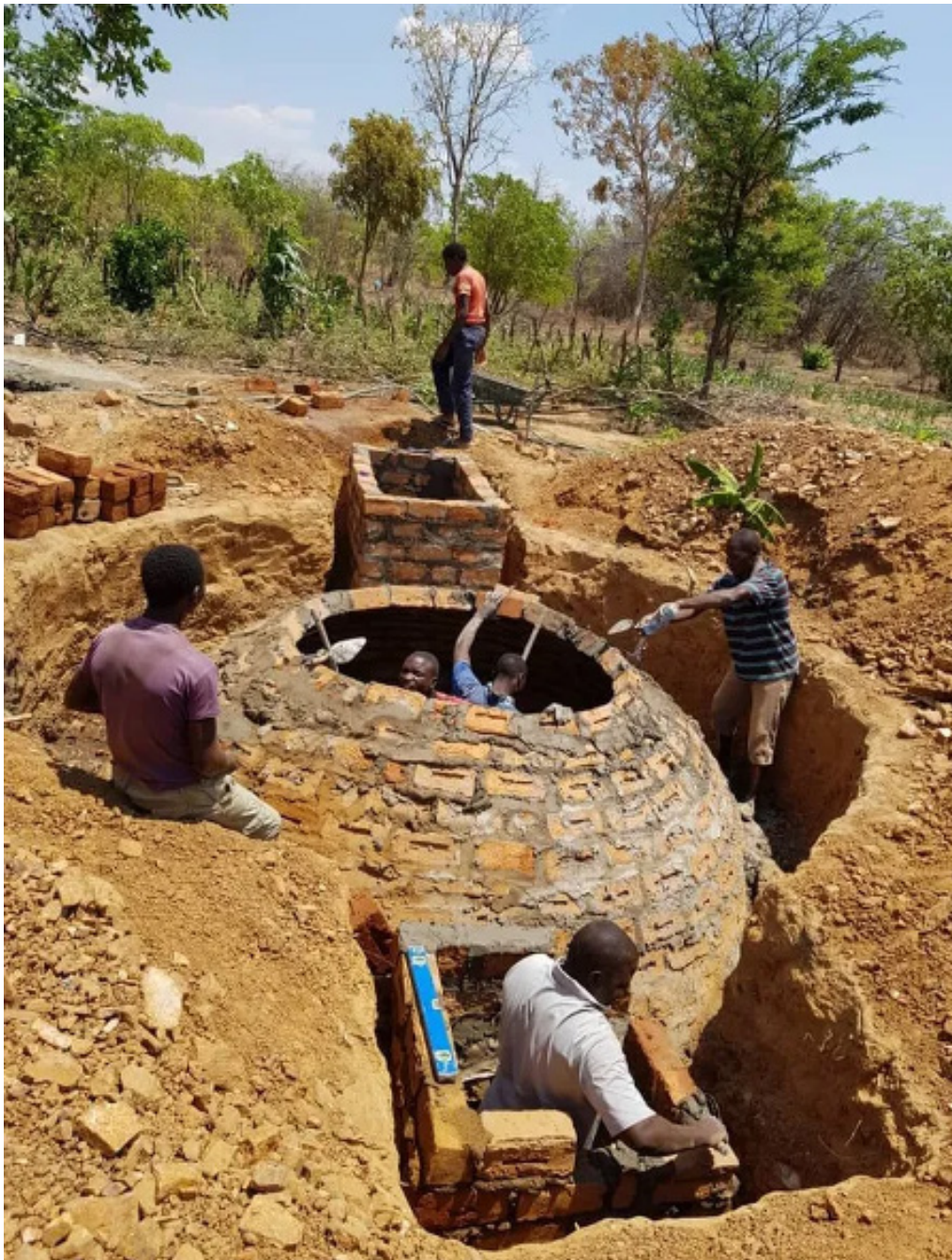
Figure VI. 1 Construction of a biogas digester in Zambia
