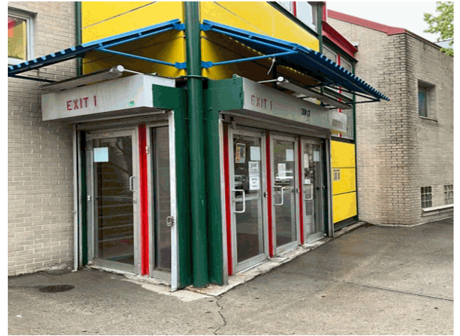
Facades A - Mapes Avenue
