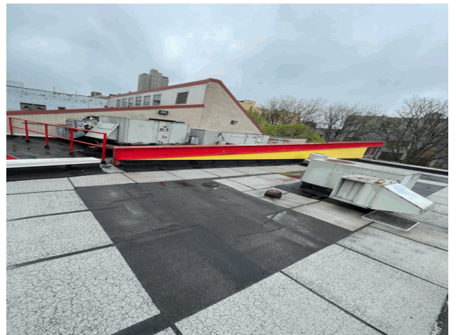
Roof 6 - Northeast View
