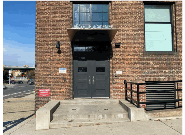
Facade A - Lafayette Avenue
