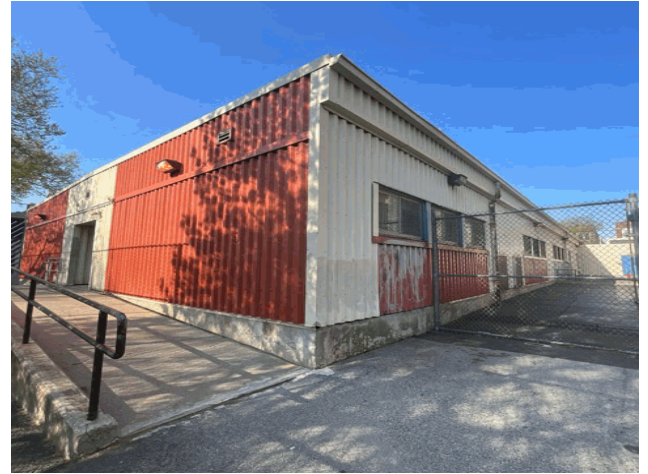
Manor Avenue - Southwest View
