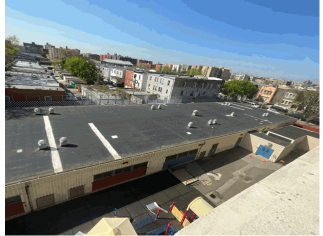
Manor Avenue - Southwest View
