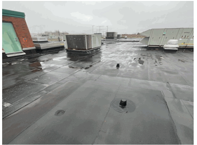
Roof 1 - West View
