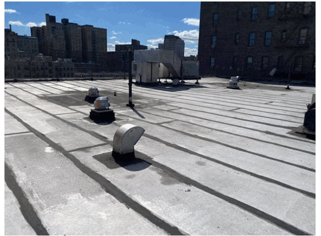
Roof 1 - Southeast View
