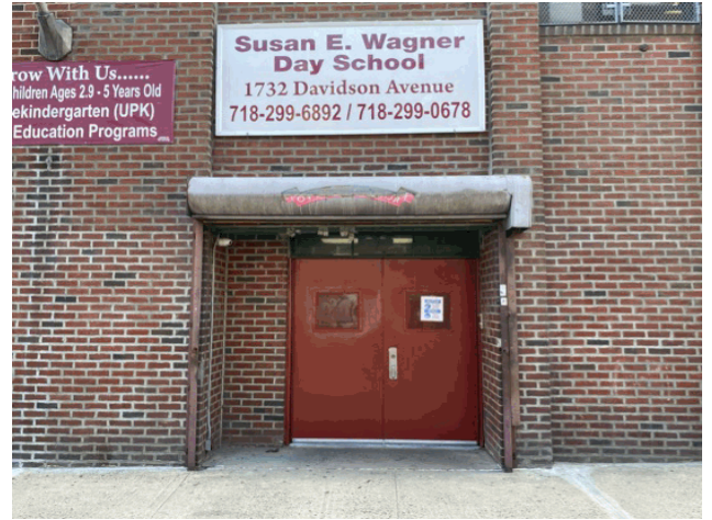
Facade A - Davidson Avenue
