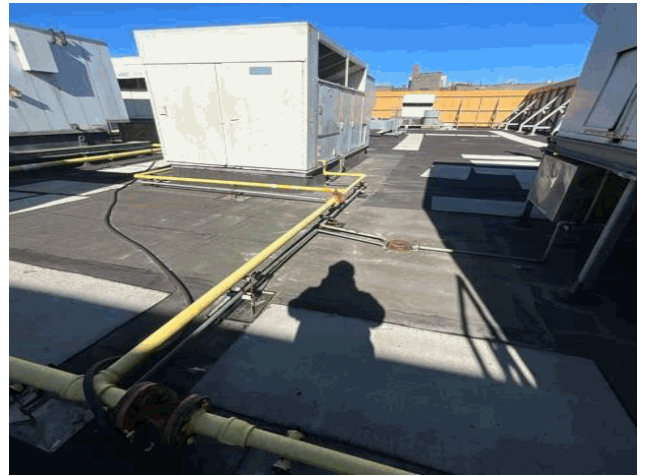
Roof 1 -North View
