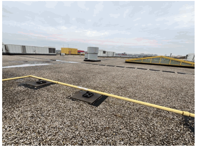
Roof 1 - Northwest View
