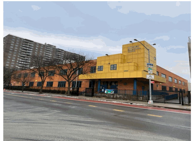
Story Avenue - Southeast View
