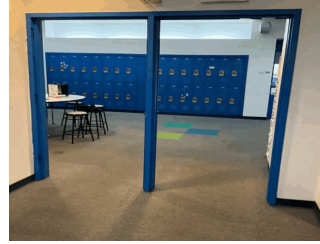
Corridor near Room 136
