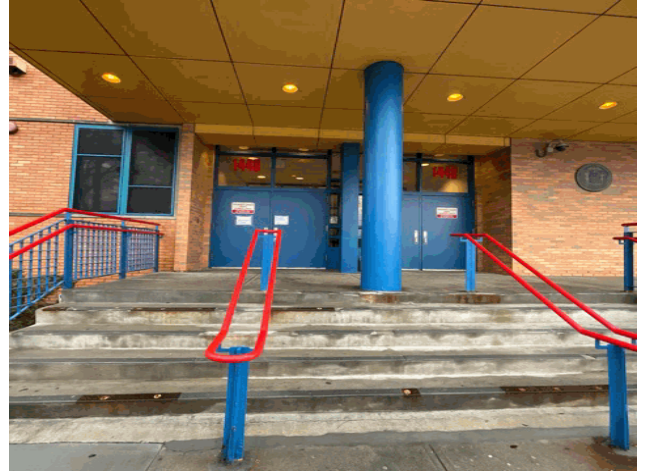
Facade A - Story Avenue
