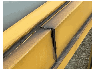
Skylight SK frame
