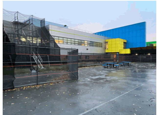
Facade A - Bathgate Avenue
