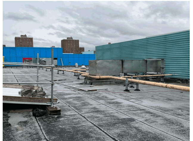
Roof 1 - Southwest View
