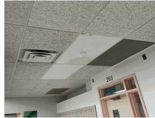
Corridor near Room 263
