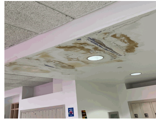
Corridor near Room 207
