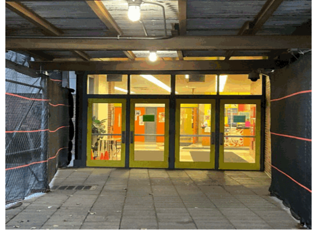
Facade A - Bathgate Avenue
