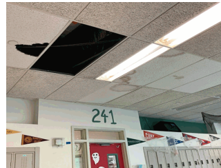
Corridor near Room 241
