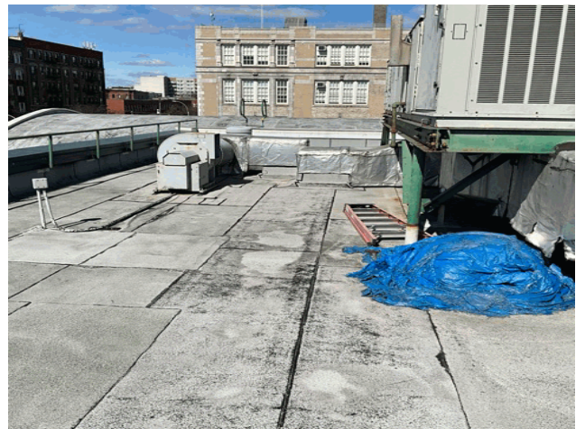
Roof 1 - West View
