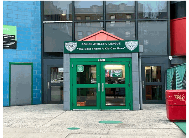
Facade A - Longwood Avenue
