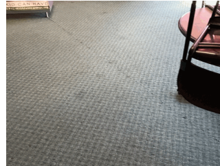
2nd Floor lobby
