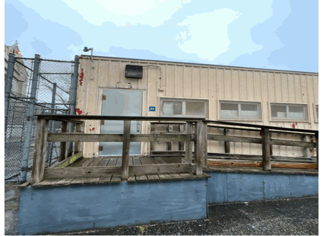
T1 - Facade A
