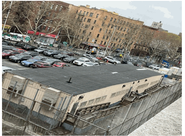
Roof 2 - North View from Main Asset X400
