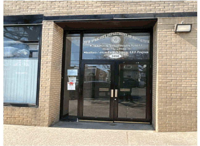
Facade A - East Tremont Avenue
