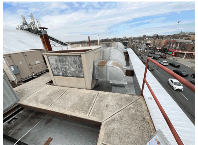
Roof 1 - Northwest View
