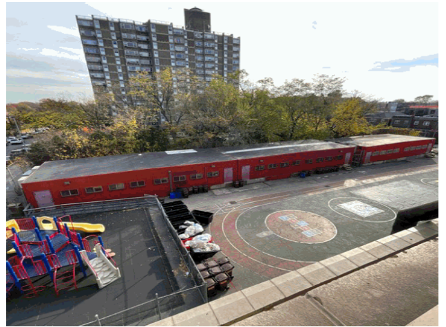
Roof 1 - Northeast View
