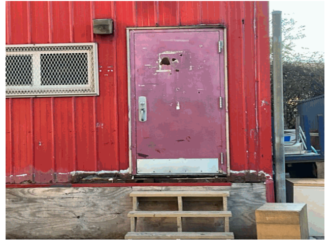
Facade A - Facade Facing Main Asset
