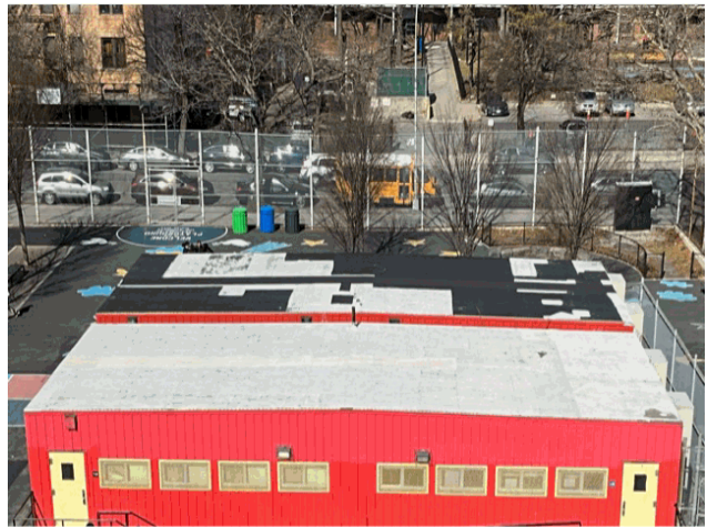
Roof 1 - West View
