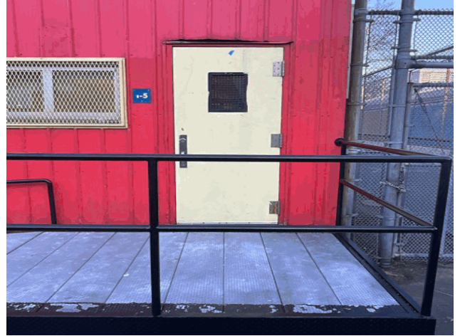
Facade A - Unit T5 Northwest View
