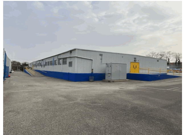
Crawford Avenue - East View
