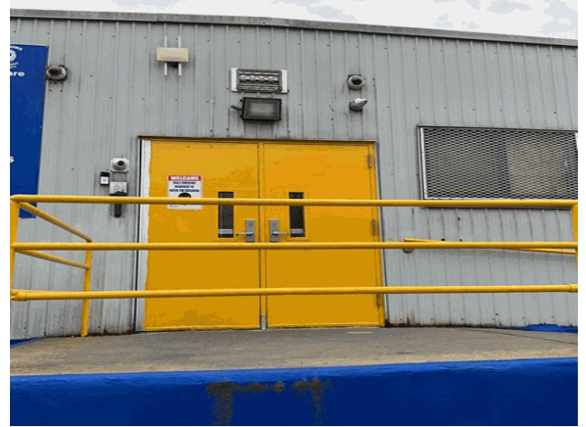
Facade A - Crawford Avenue
