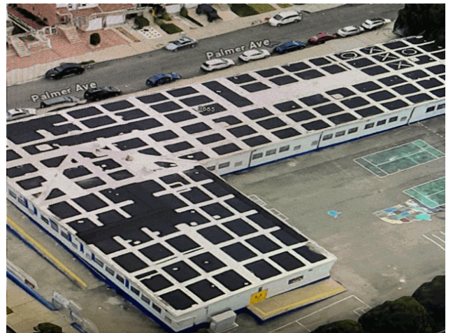
Roof 1 - Aerial View (from Google Earth)
