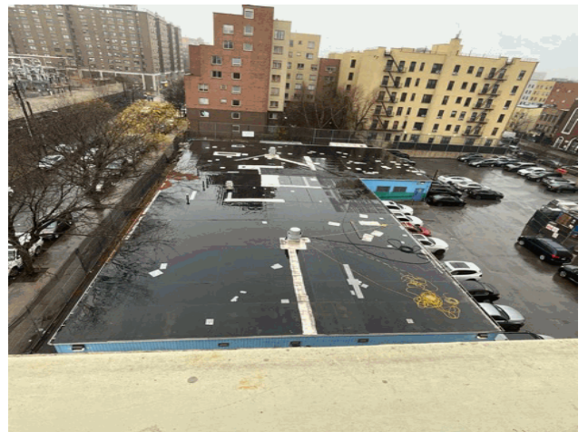
Roof 1 - Northwest View from Main Asset X118
