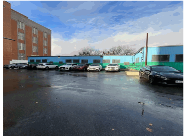
Facade D, E and F - North View
