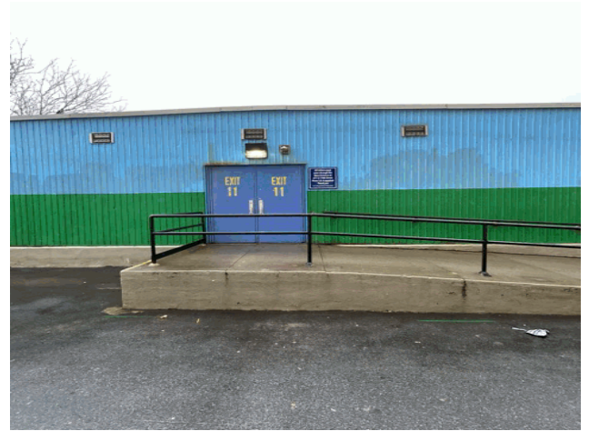
Facade A - Schooyard
